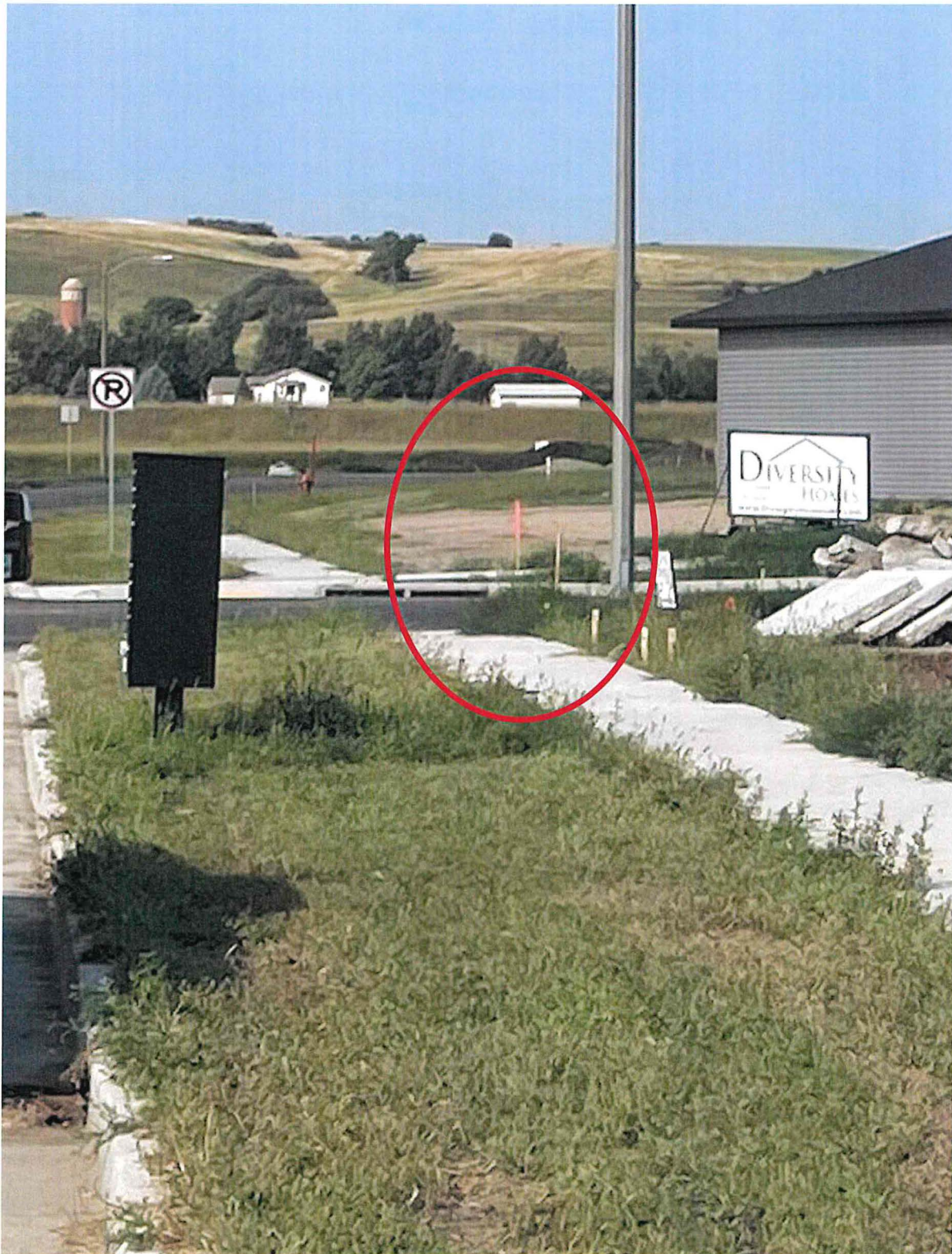
Photo 3: Stop sign not yet installed. The red circle shows lath stake painted pink is marking location of where the stop sign is to be installed.
