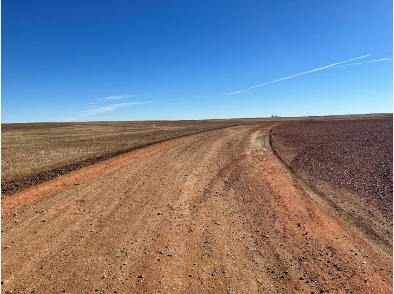
Figure 9 – Landfill Access Road, Scranton Equity Exchange
