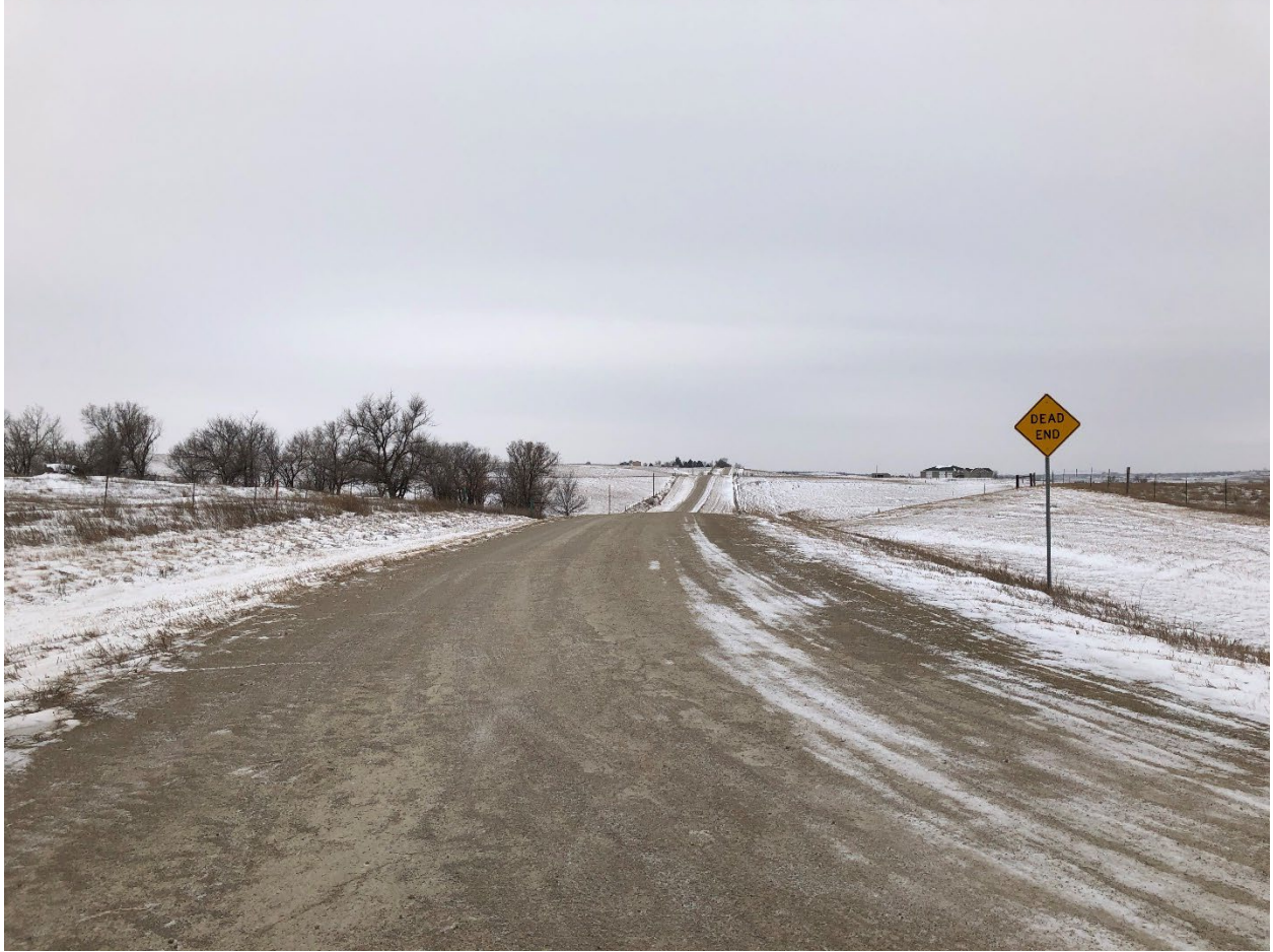
Figure 5 – 38 th St SW, Stark County Right of Way
