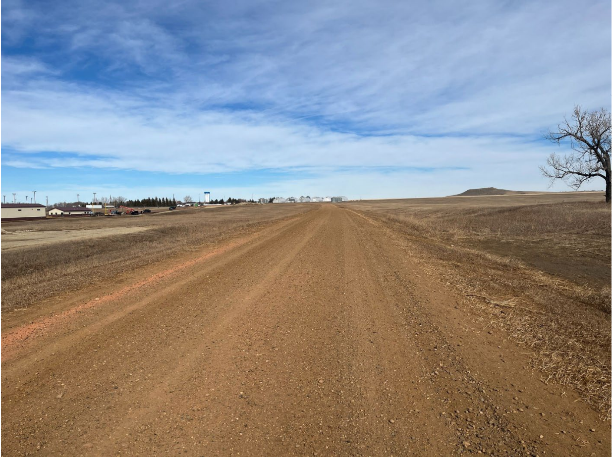
Figure 19 – Landfill Access Road, Scranton Equity Exchange
