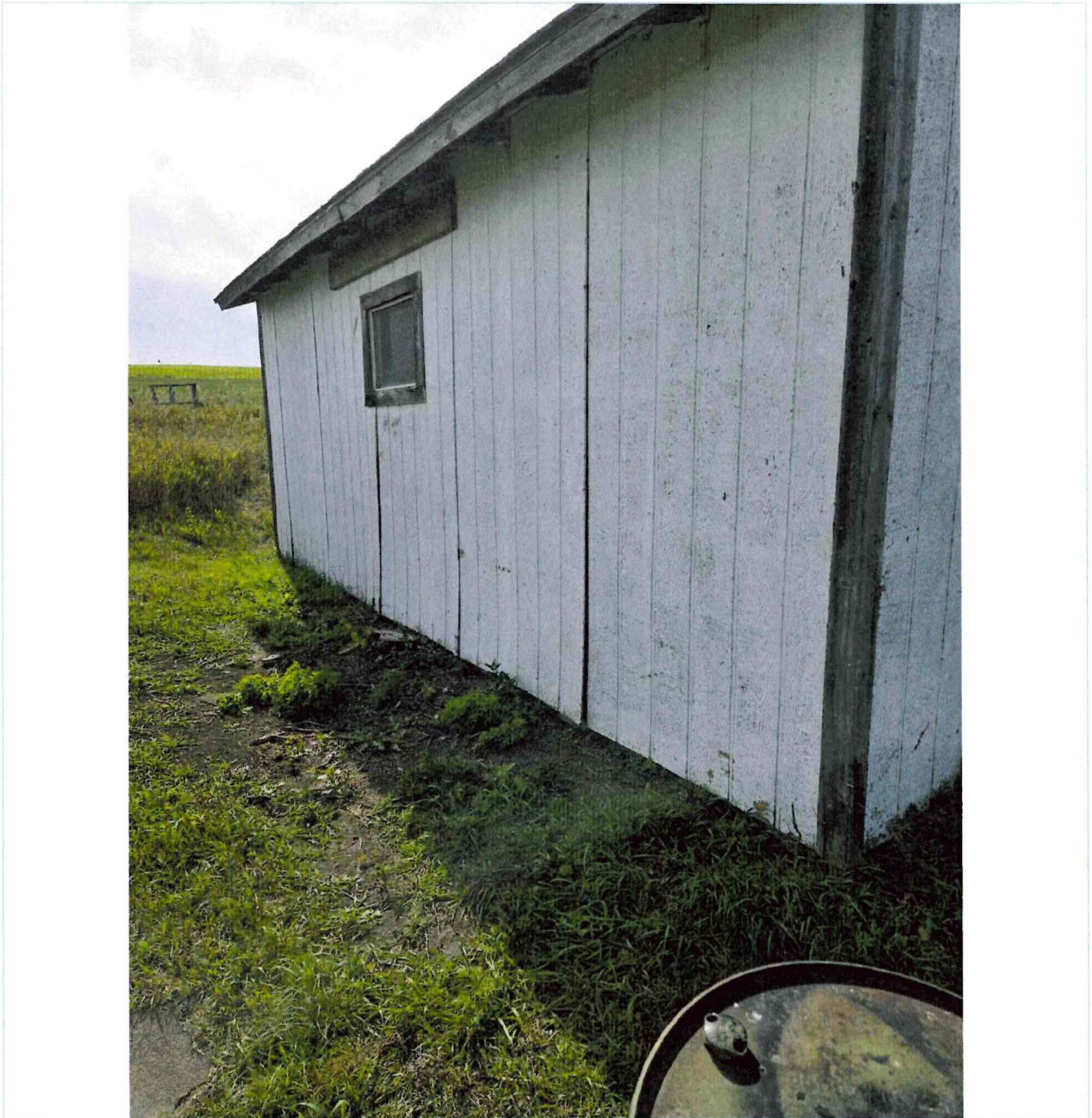
(P8) White garage – east side
