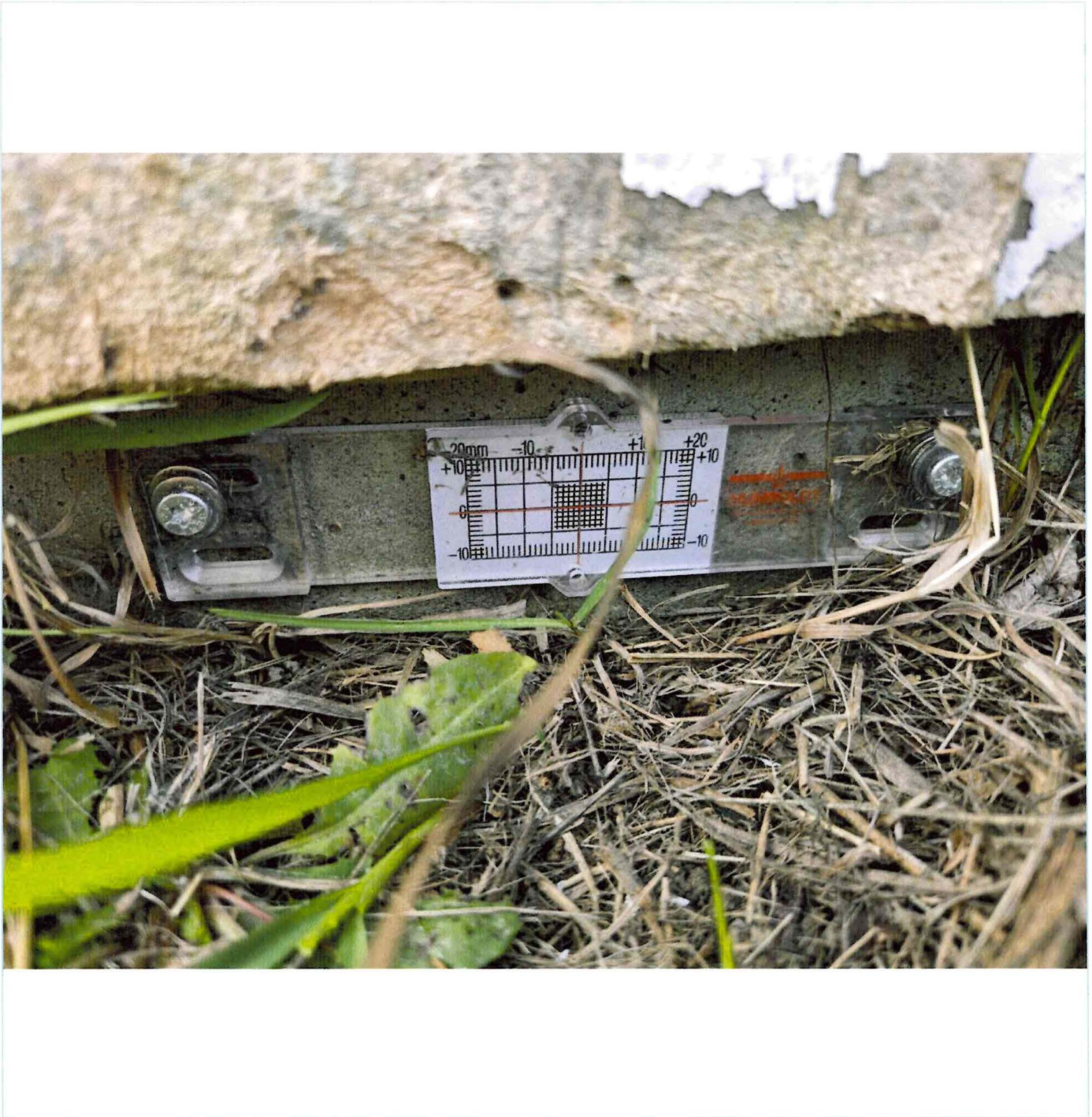
(P7) White garage – east side
