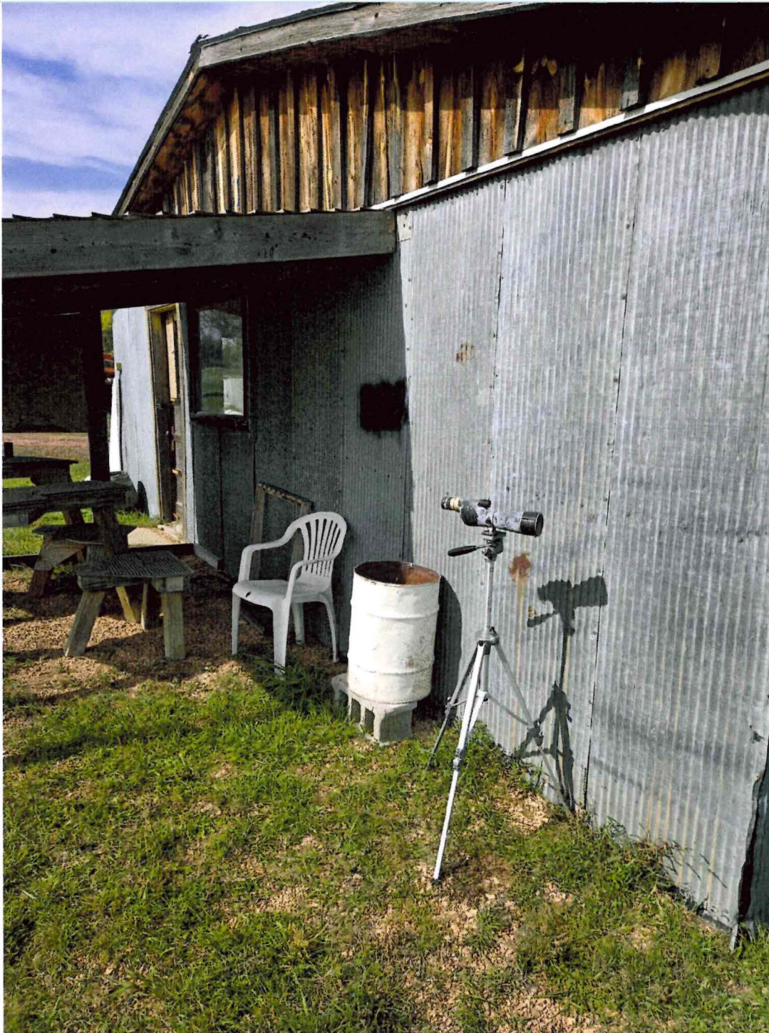
(P11) Gray shed – south side
