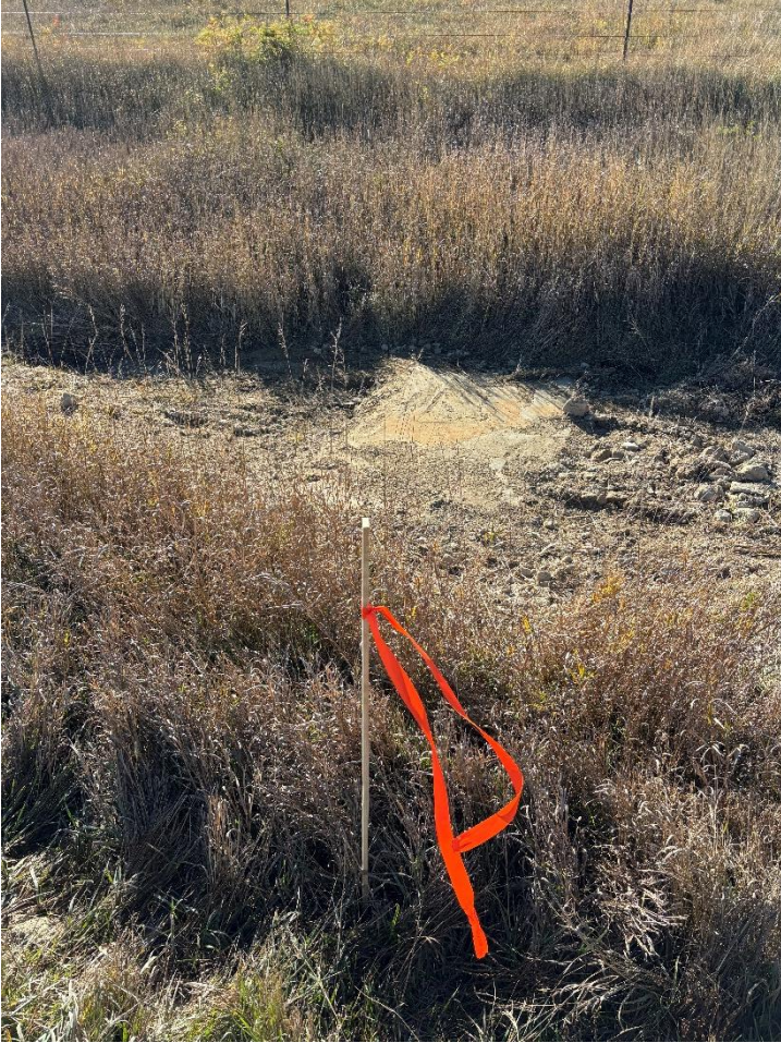
Figures 6 & 7 - Excess grout was also found in the ditch in the PSC's follow-up inspection.
