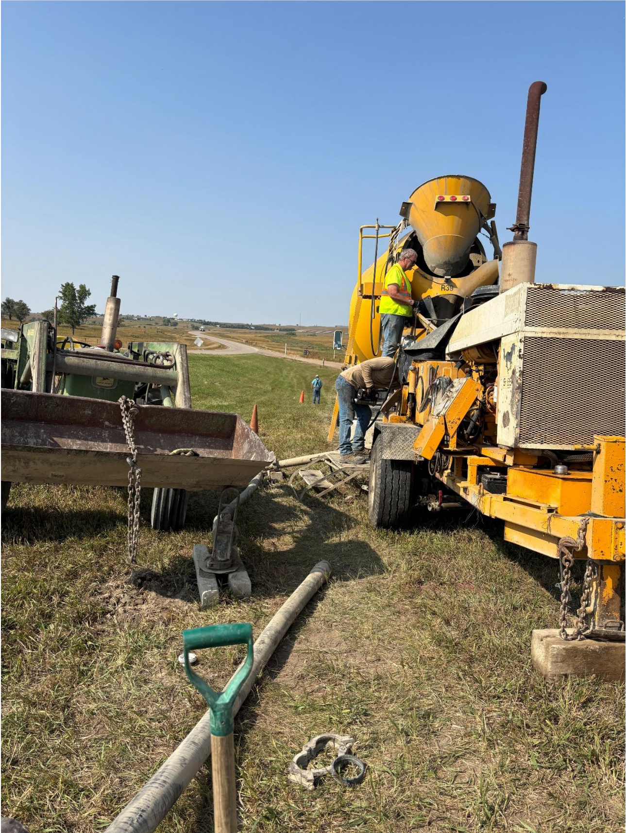
Figure 6: Pumping grout along Lehigh Road near Dickinson
