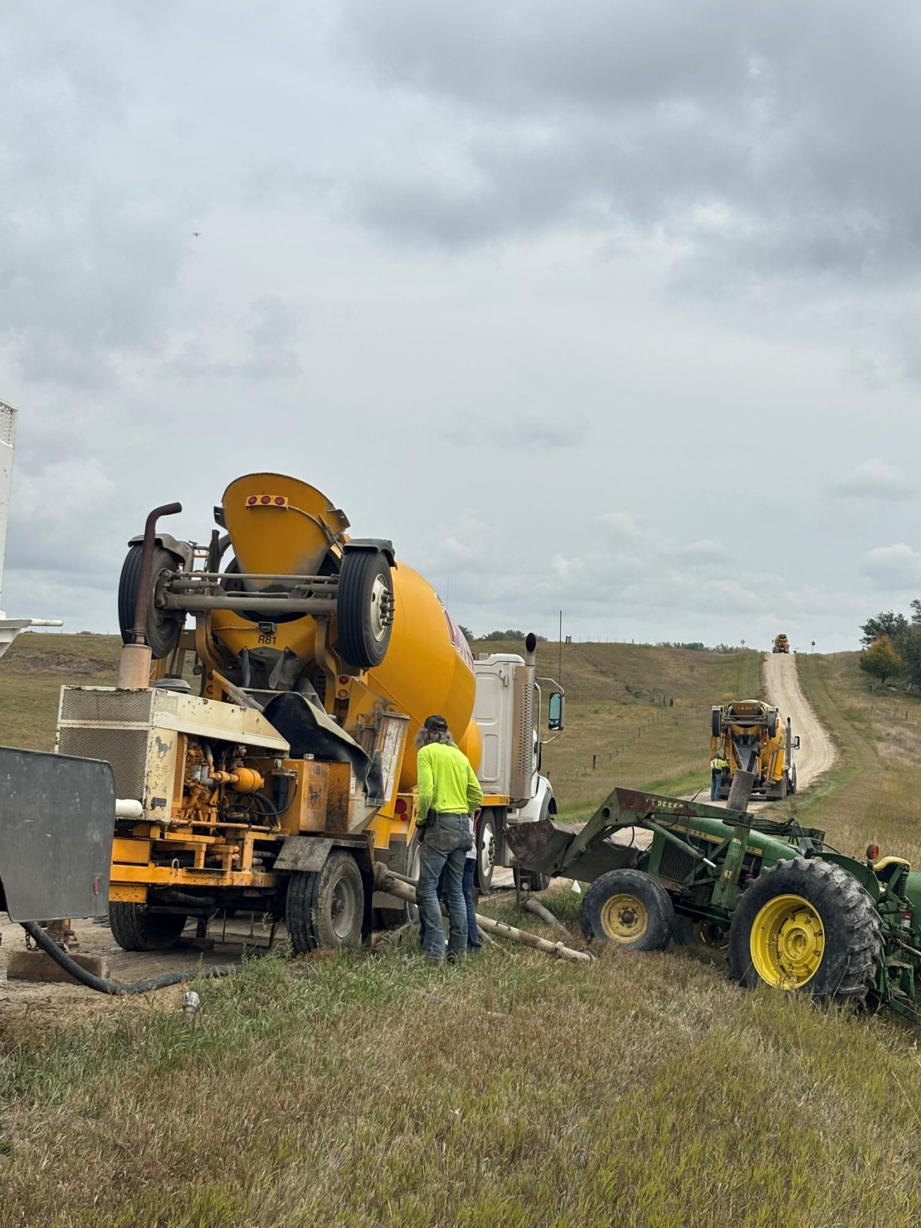
Figure 5: Pumping grout along 38 th Street SW near Dickinson
