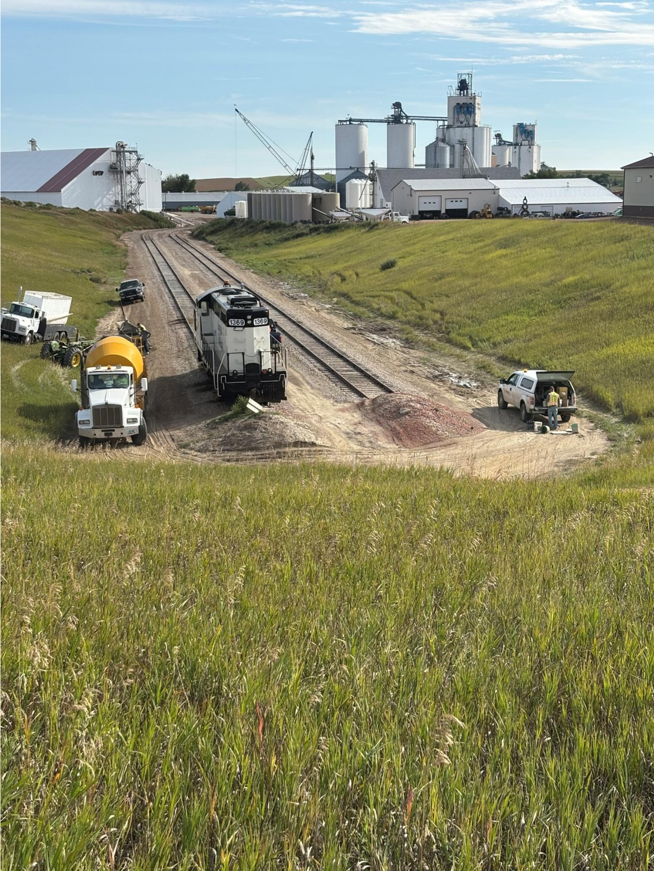
Figure 3: Pumping grout alongside Scranton Equity Exchange’s rail spur
