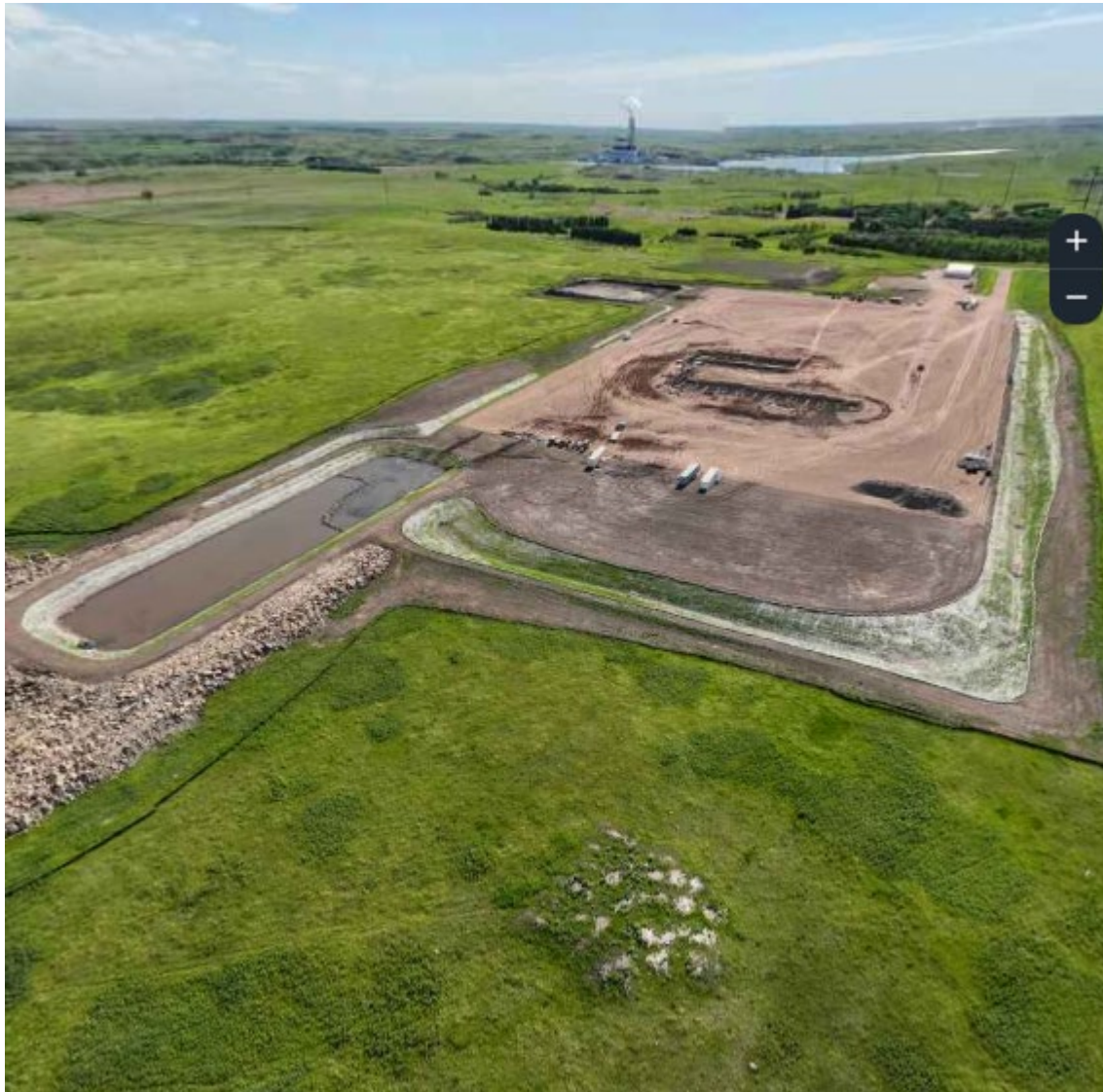
Photo 1: East Oliver HVDC Converter Station Civil Work
