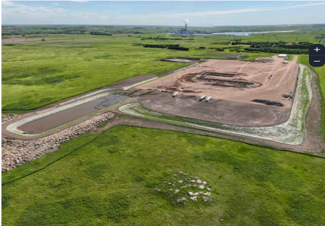
Photo 1: East Oliver HVDC Converter Station Civil Work
