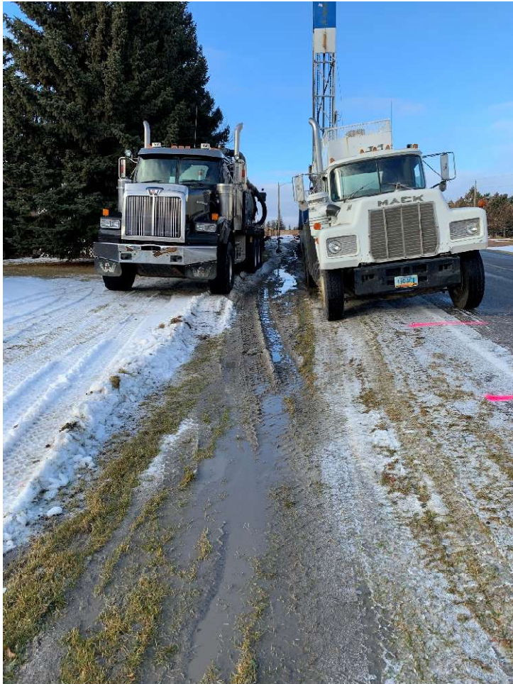
Figure 4 Looking West from N 10th St. Notice no yellow pin flags or paint.
