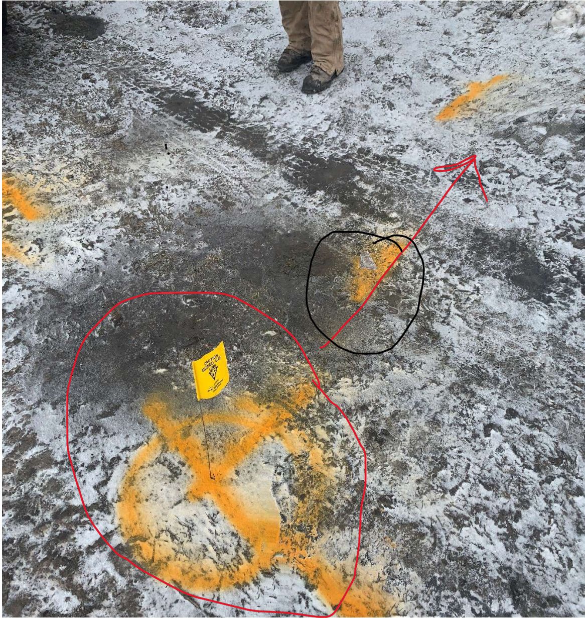
Figure 8 This how a service line take off is marked. The red circle is the location of the tap, and the red arrow is the direction of the gas service line to the resident. The outer black circle is where the drill hole was drilled.
