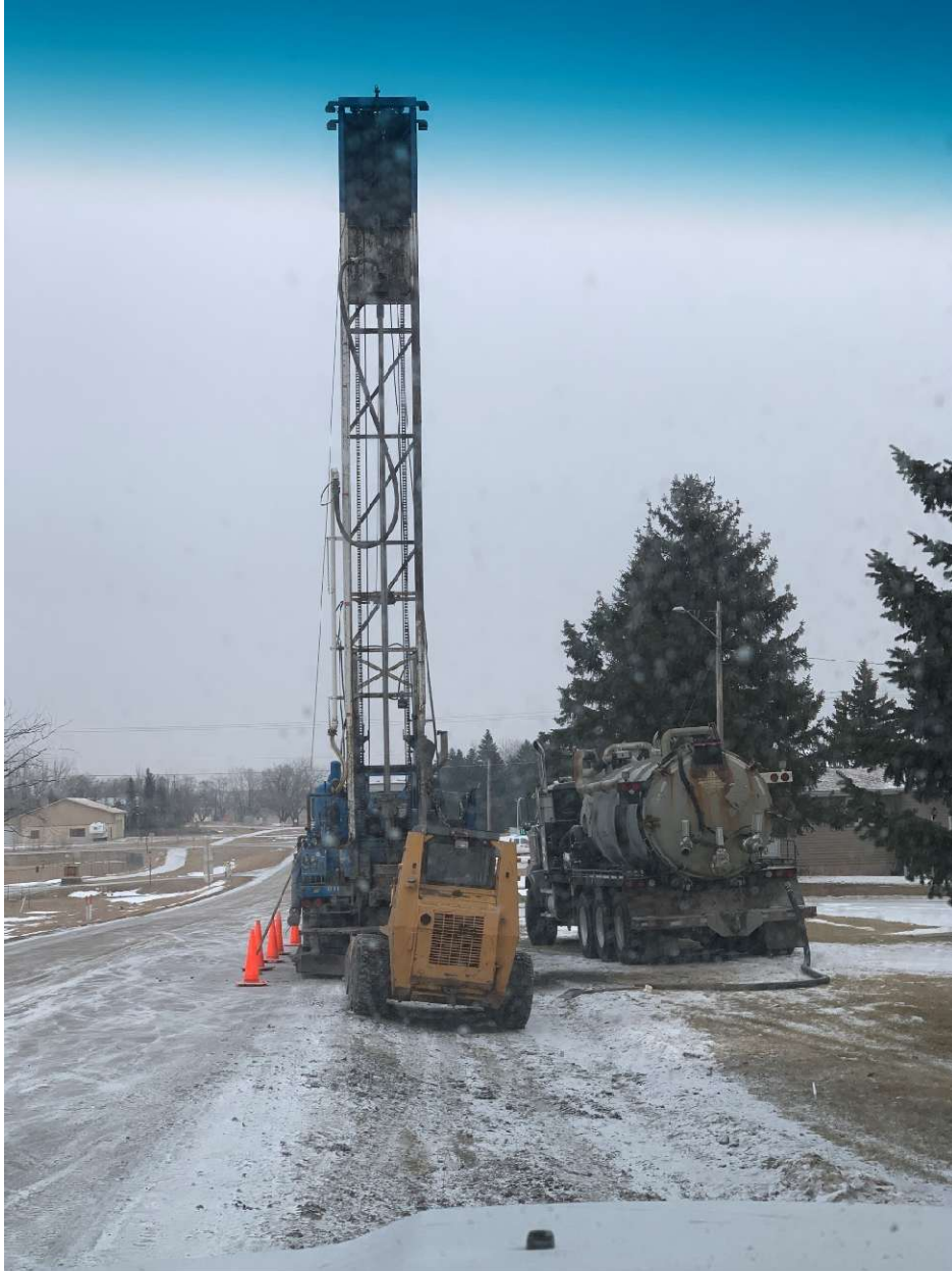
Figure 5 The crew drilling the morning at approximately 9:00 am.
