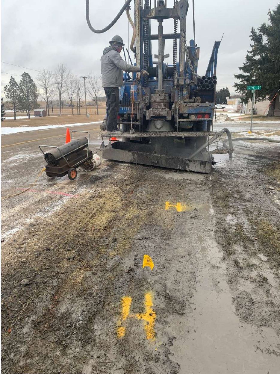
Figure 7 Corner of Hwy 10 and N 10 th St. facing East.
