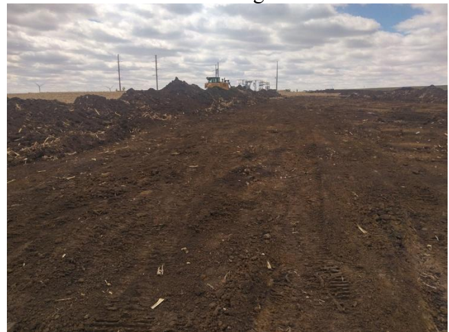
Site 2 Looking South
