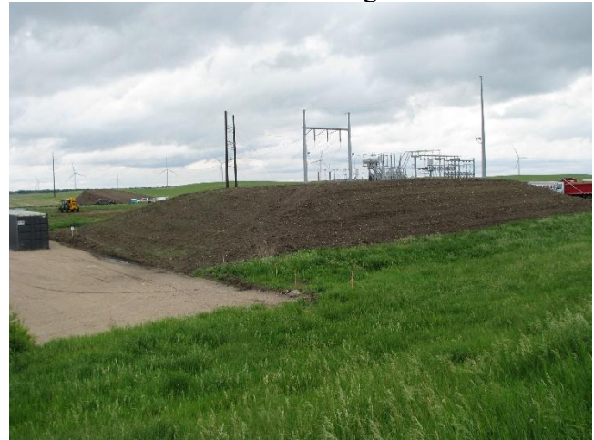
View of Site 1 Looking Southeast
