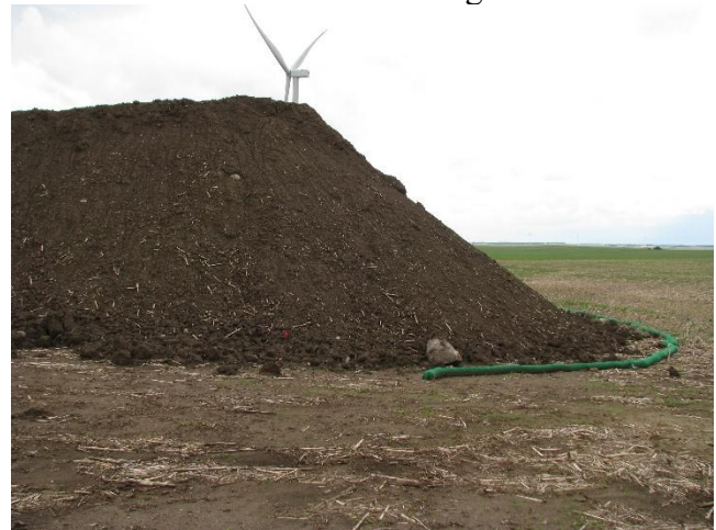
View of Site 2 Looking North
