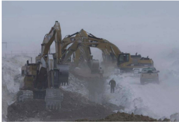
1 Figure 1 Typical Winter Pipeline Installation.
