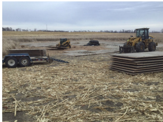
Figure 4 Installation of Structure Work Pad
