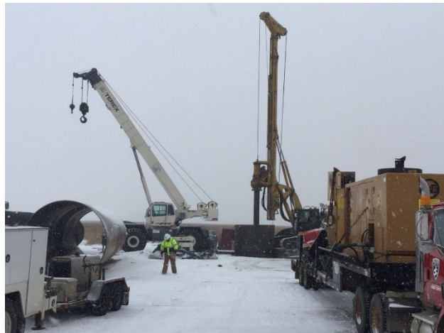
Figure 2 Typical Winter Drilled Pier Foundation Installation.
