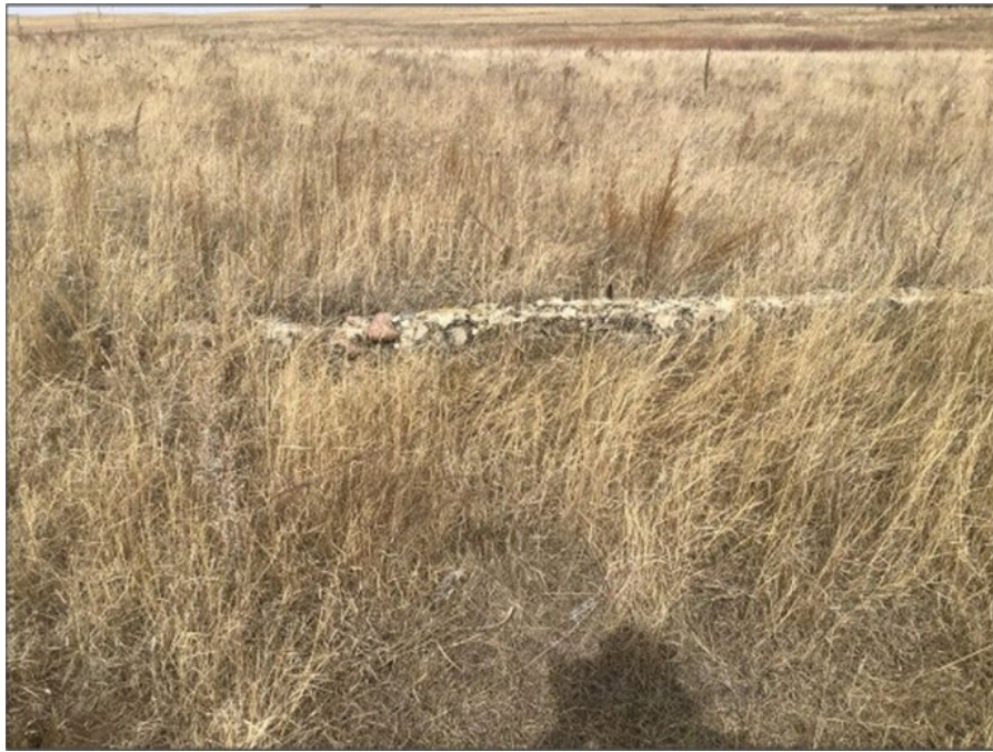
Photo 4.3-1. View of Feature 1, Concrete Foundation, View West, Site 32MO1721.
