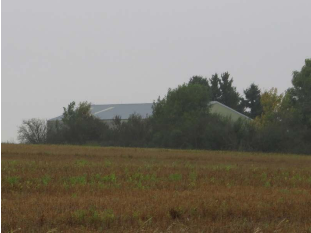
HS-KS-047. 15074 71st St NW, Grenora, Williams County, North Dakota. Property overview. View to the Southwest. Photo Number 0650. (Tetra Tech 2025).
