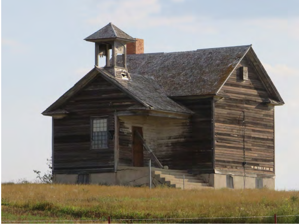
32WIX2197. Haug School.15211 71st St NW, Grenora, Williams County, North Dakota. F01. View to the Northeast. Photo Number 0222. (Tetra Tech 2025).
