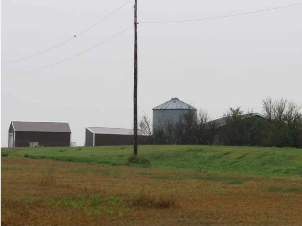
HS-KS-047. 15074 71st St NW, Grenora, Williams County, North Dakota. Property overview. View to the Southwest. Photo Number 0647. (Tetra Tech 2025).
