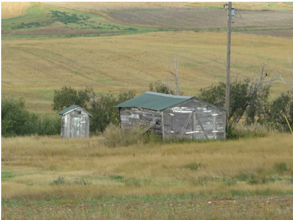
HS-KS-027. 150th Ave NW, Williston, Williams County, North Dakota. Property overview. View to the Northwest. Photo Number 0354. (Tetra Tech 2025).
