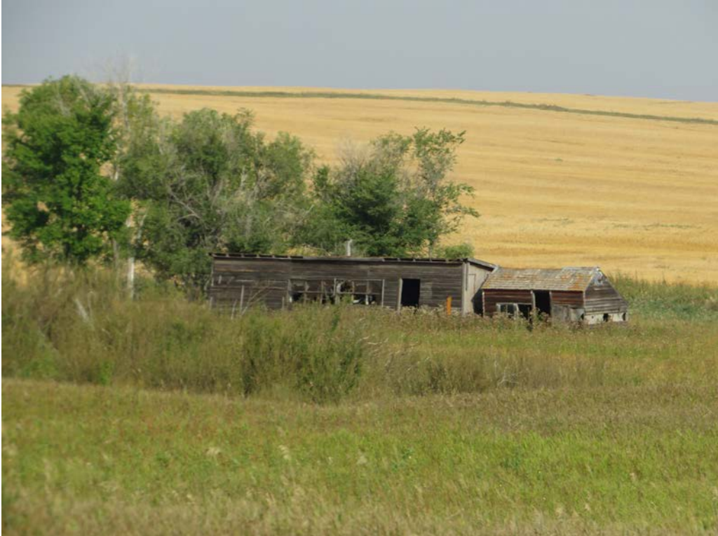
HS-KS-025. 65th St NW, Williston, Williams County, North Dakota. Property overview. View to the Northwest. Photo Number 0313. (Tetra Tech 2025).
