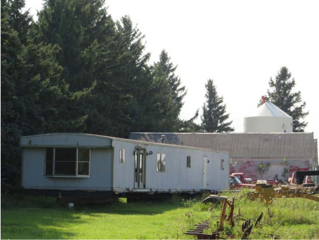
HS-KS-033. 14710 74th st NW, Grenora, Williams County, North Dakota. Property overview. View to the South. Photo Number 0459. (Tetra Tech 2025).
