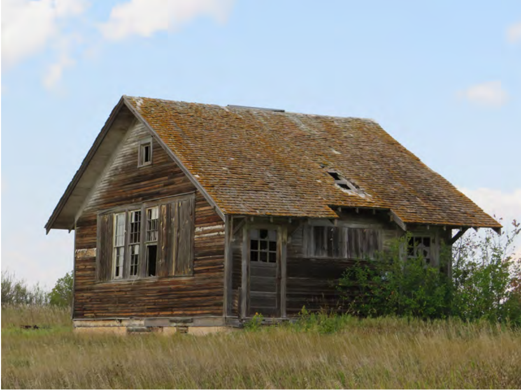
32WIX2458. Eureka Number 2 School.7671-7681 143rd Ave NW, Zahl, Williams County, North Dakota. F01. View to the North-west. Photo Number 0552. (Tetra Tech 2025).
