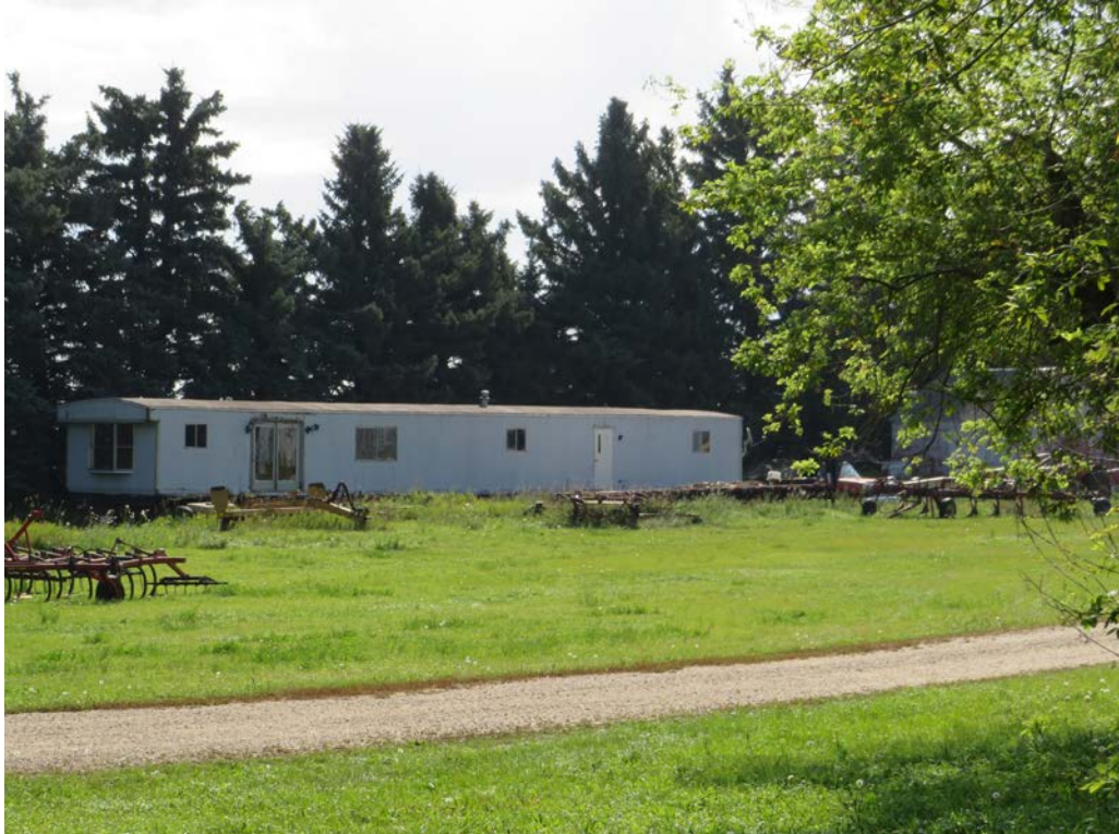
HS-KS-033. 14710 74th st NW, Grenora, Williams County, North Dakota. Property overview. View to the Southwest. Photo Number 0452. (Tetra Tech 2025).
