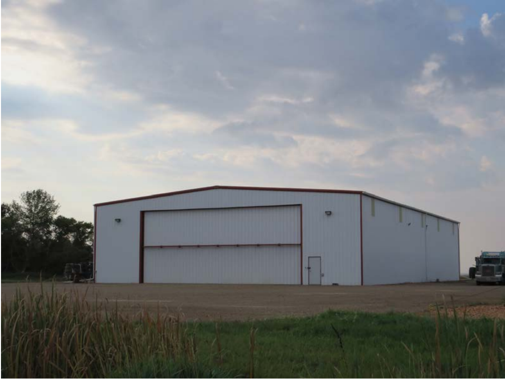
HS-KS-020. 15086 68th St NW, Williston, Williams County, North Dakota. Property overview. View to the Southeast. Photo Number 0243. (Tetra Tech 2025).
