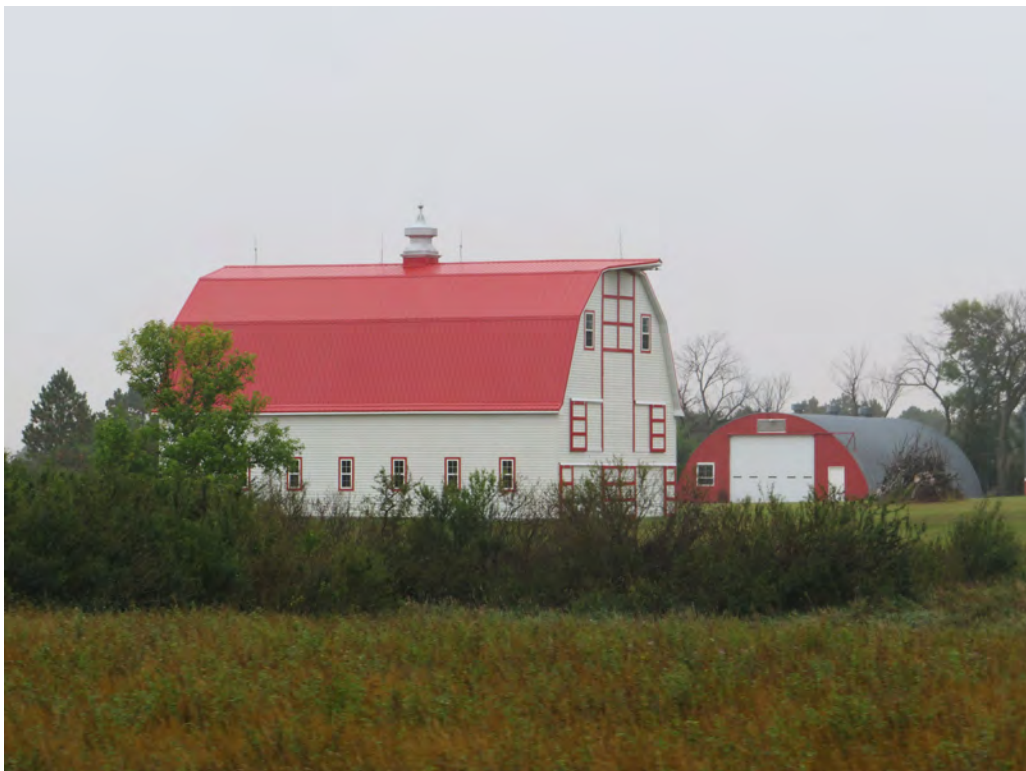
32WIX933. 14803 72nd St NW, Grenora, Williams County, North Dakota. F02 (left) and F04 (right). View to the Northwest. Photo Number 0622. (Tetra Tech 2025).
