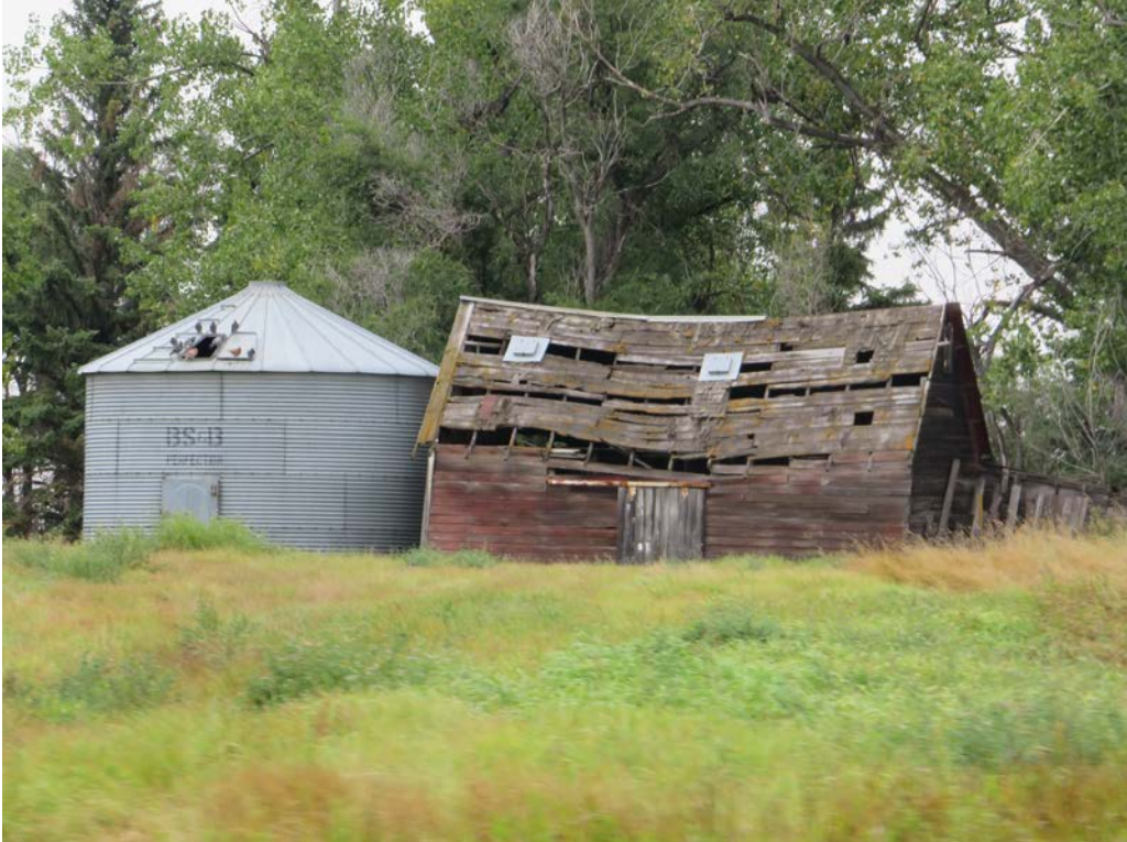
HS-KS-061. 14581 69th St NW, Williston, Williams County, North Dakota. Property overview. View to the North. Photo Number 0778. (Tetra Tech 2025).
