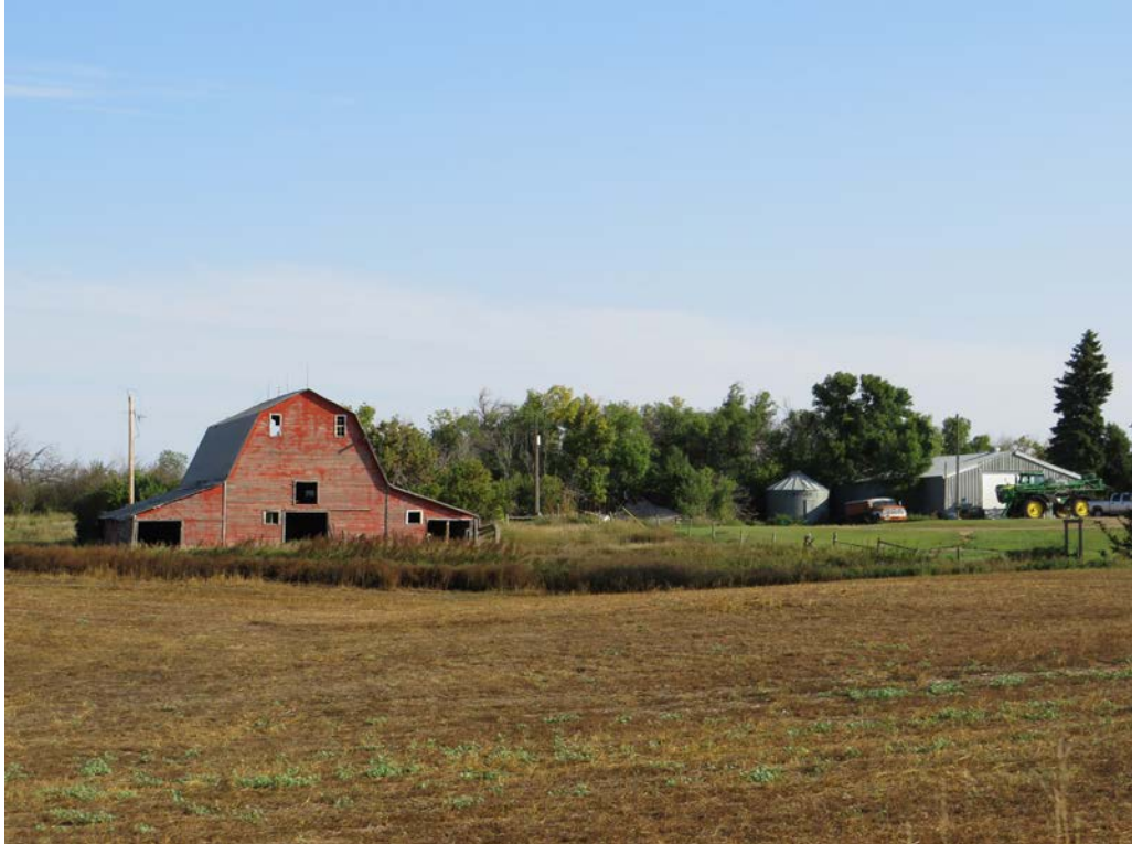
HS-KS-001. 67th St NW, Williston, Williams County, North Dakota. Property overview. View to the Northeast. Photo Number 0012. (Tetra Tech 2025).
