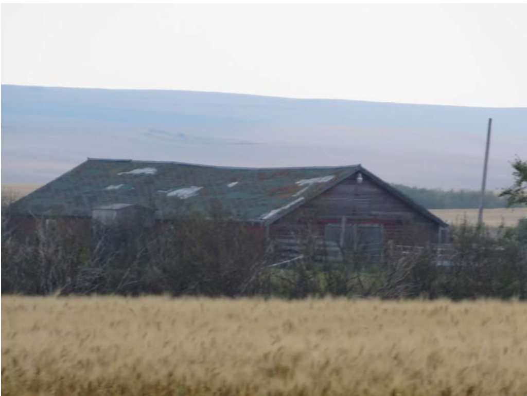
HS-KS-028. 14802 - 14788 67 th St NW, Williston, Williams County, North Dakota. Property overview. View to the Southeast. Photo Number 0364. (Tetra Tech 2025).
