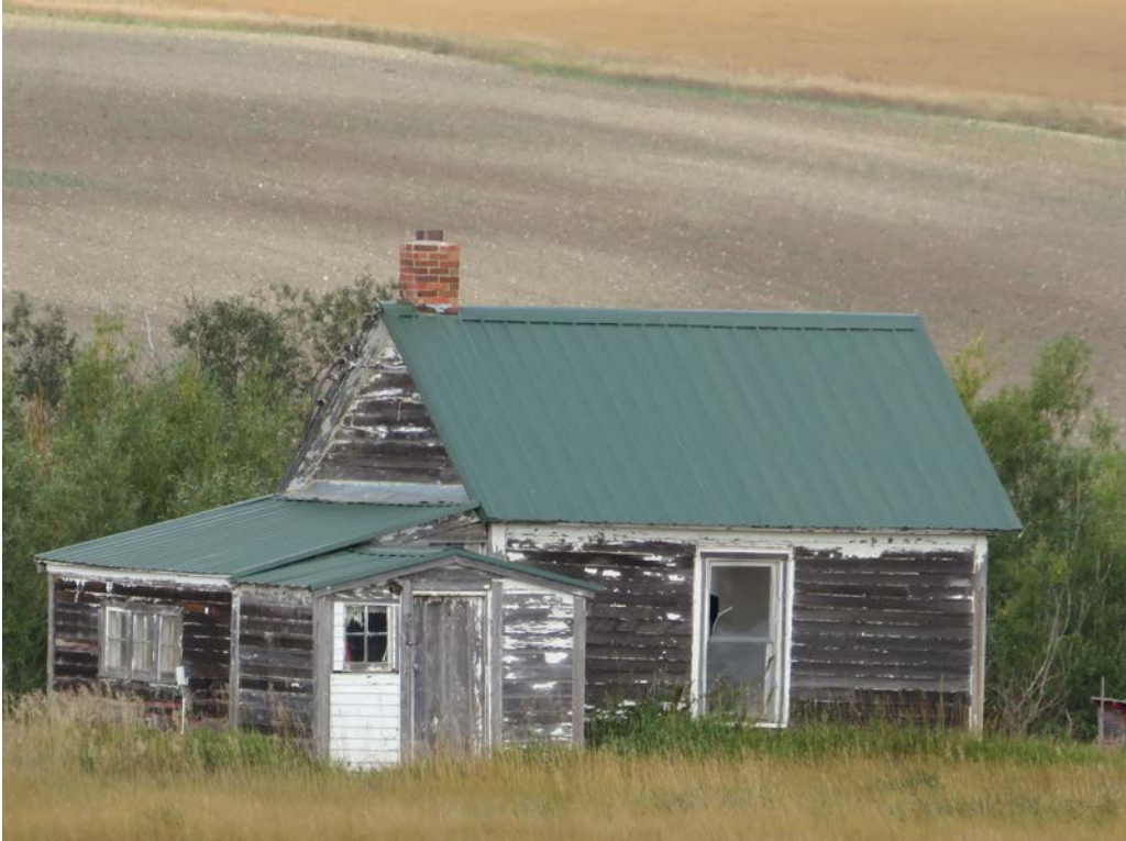
HS-KS-027. 150th Ave NW, Williston, Williams County, North Dakota. Property overview. View to the Northwest. Photo Number 0356. (Tetra Tech 2025).
