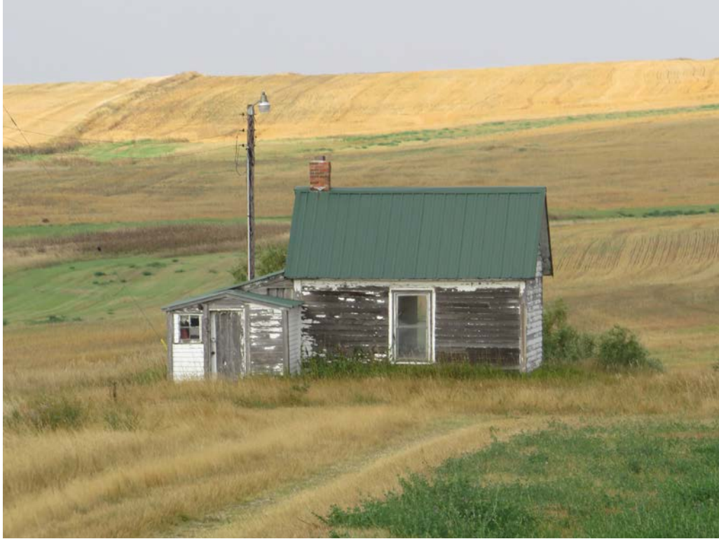
HS-KS-027. 150th Ave NW, Williston, Williams County, North Dakota. Property overview. View to the Southwest. Photo Number 0346. (Tetra Tech 2025).
