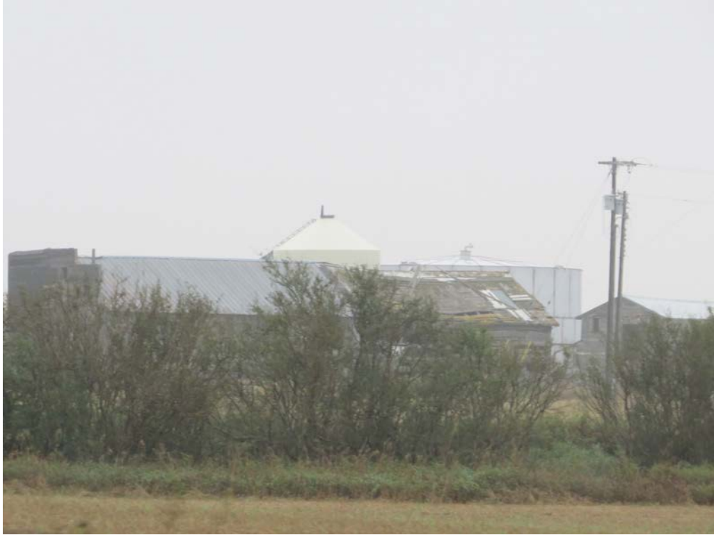
HS-KS-044. 14740 72nd St NW, Grenora, Williams County, North Dakota. Property overview. View to the Southwest. Photo Number 0607. (Tetra Tech 2025).
