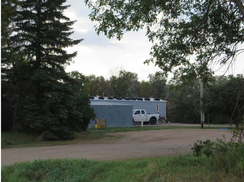
HS-KS-020. 15086 68th St NW, Williston, Williams County, North Dakota. Property overview. View to the Southeast. Photo Number 0246. (Tetra Tech 2025).
