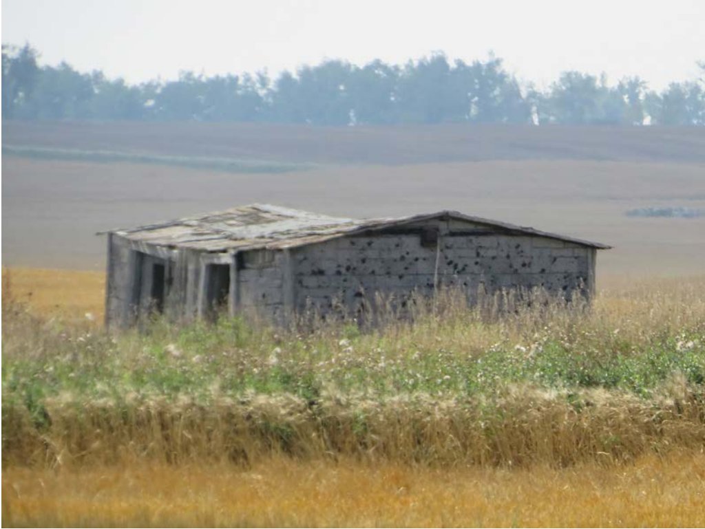
HS-KS-039. 76th St NW, Grenora, Williams County, North Dakota. Property overview. View to the Southwest. Photo Number 0545. (Tetra Tech 2025).
