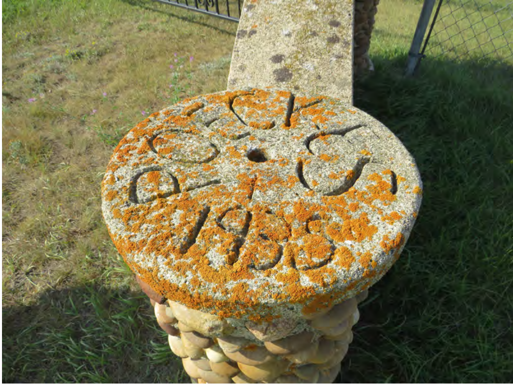
32WI2589. 14908 74th St NW, Grenora, Williams County, North Dakota. F01 pillar cap. View to the South. Photo Number 0421. (Tetra Tech 2025).
