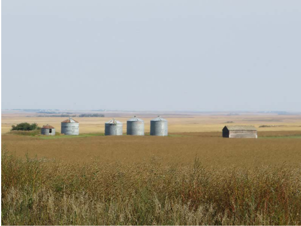
HS-KS-010. 147th Ave NW, Williston, Williams County, North Dakota. Property overview. View to the Northeast. Photo Number 0128. (Tetra Tech 2025).
