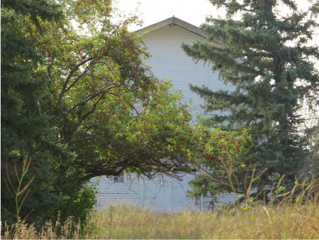
32WIX932. 14606 74th St NW, Grenora, Williams County, North Dakota. F02. View to the South. Photo Number 0465. (Tetra Tech 2025).
