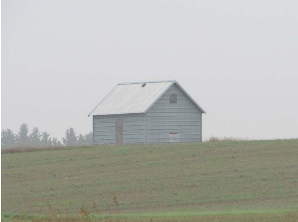
HS-KS-049. 150th Ave NW, Grenora, Williams County, North Dakota. Property overview. View to the Northeast. Photo Number 0655. (Tetra Tech 2025).
