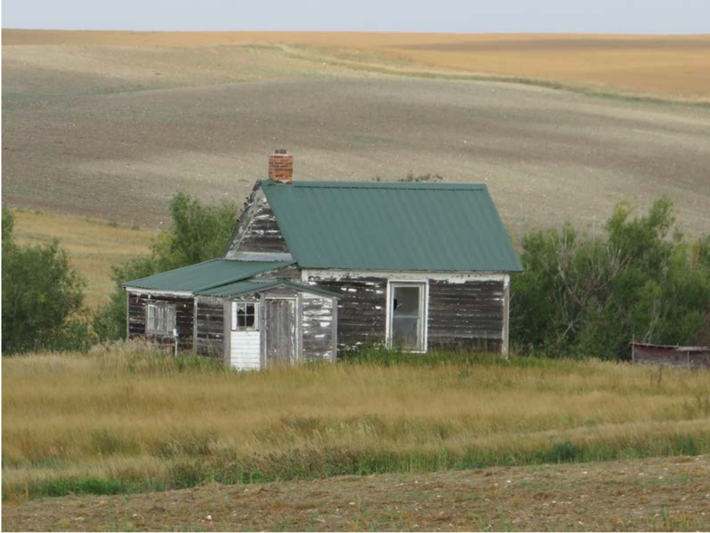
HS-KS-027. 150th Ave NW, Williston, Williams County, North Dakota. Property overview. View to the Northwest. Photo Number 0355. (Tetra Tech 2025).
