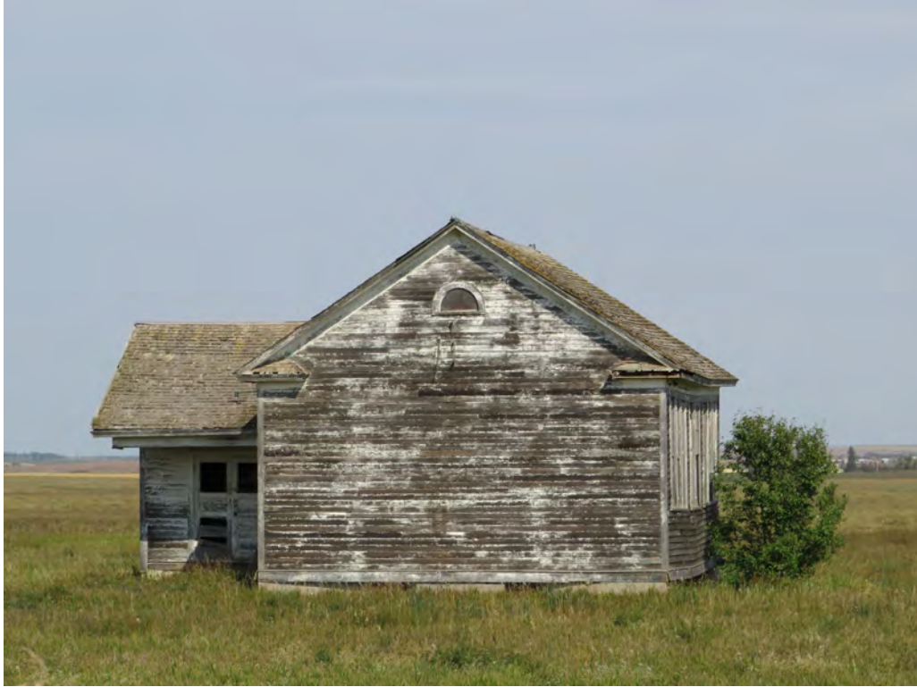
32WIX2460. Thull School.14704 75th St NW, Grenora, Williams County, North Dakota. F01. View to the North. Photo Number 0167. (Tetra Tech 2025).
