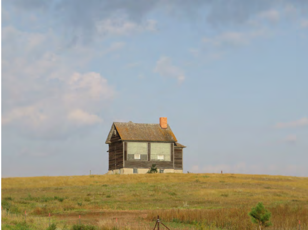
32WIX2197. Haug School.15211 71st St NW, Grenora, Williams County, North Dakota. Property overview. View to the North-west. Photo Number 0215. (Tetra Tech 2025).
