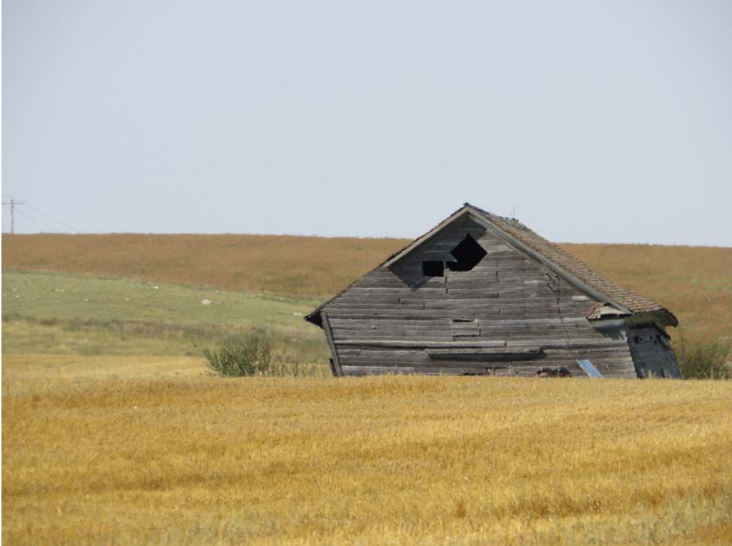
HS-KS-011. 7609 147th Ave NW, Grenora, Williams County, North Dakota. Property overview. View to the Southwest. Photo Number 0144. (Tetra Tech 2025).
