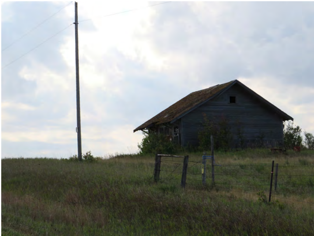
32WIX2458. Eureka Number 2 School.7671-7681 143rd Ave NW, Zahl, Williams County, North Dakota. Property overview. View to the Southwest. Photo Number 0547. (Tetra Tech 2025).
