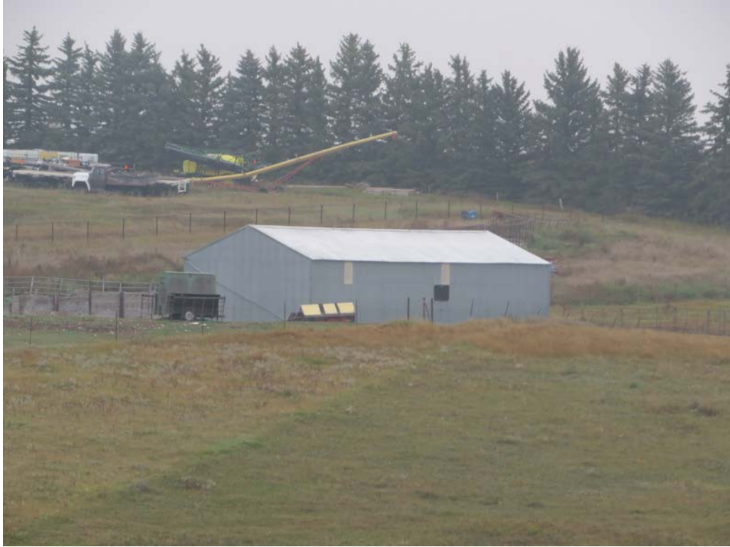
HS-KS-050. 7054 150th Ave NW, Grenora, Williams County, North Dakota. Property overview. View to the Northeast. Photo Number 0659. (Tetra Tech 2025).
