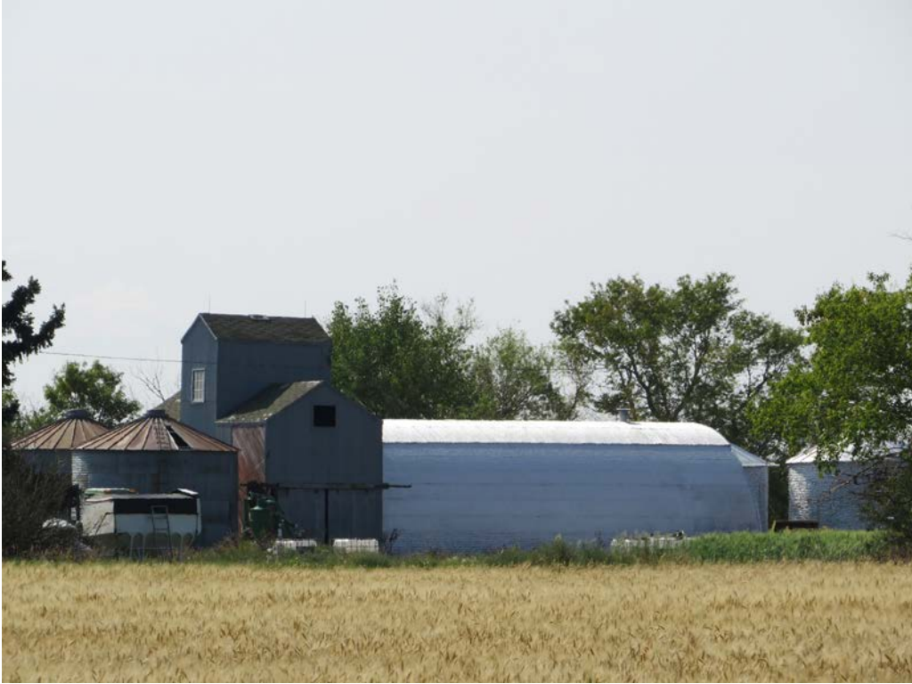
HS-KS-016. 6755 144th Ave NW, Williston, Williams County, North Dakota. Property overview. View to the Southwest. Photo Number 0201. (Tetra Tech 2025).
