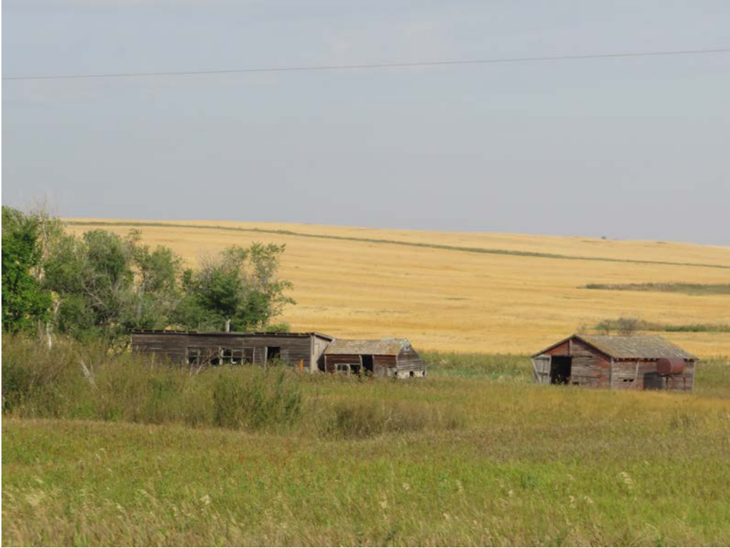
HS-KS-025. 65th St NW, Williston, Williams County, North Dakota. Property overview. View to the Northwest. Photo Number 0314. (Tetra Tech 2025).
