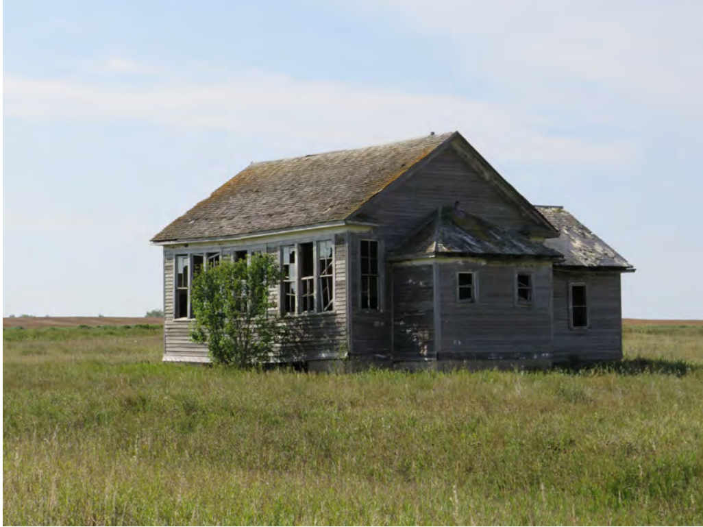
32WIX2460. Thull School.14704 75th St NW, Grenora, Williams County, North Dakota. F01. View to the Southwest. Photo Number 0160. (Tetra Tech 2025).
