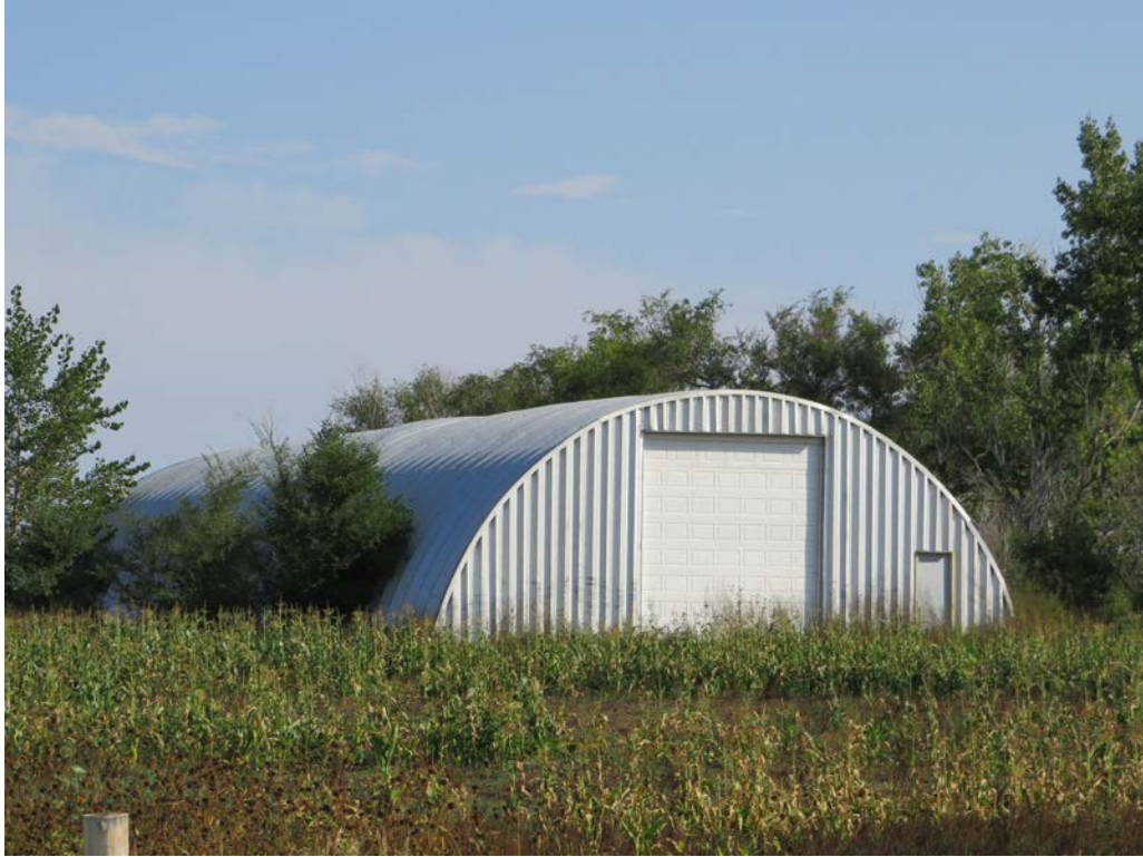
HS-KS-005. 14729 69th St NW, Williston, Williams County, North Dakota. Property overview. View to the Northwest. Photo Number 0063. (Tetra Tech 2025).
