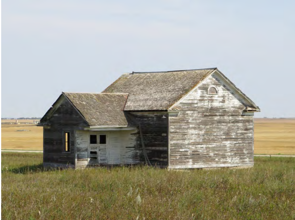
32WIX2460. Thull School.14704 75th St NW, Grenora, Williams County, North Dakota. F01. View to the Northeast. Photo Number 0170. (Tetra Tech 2025).
