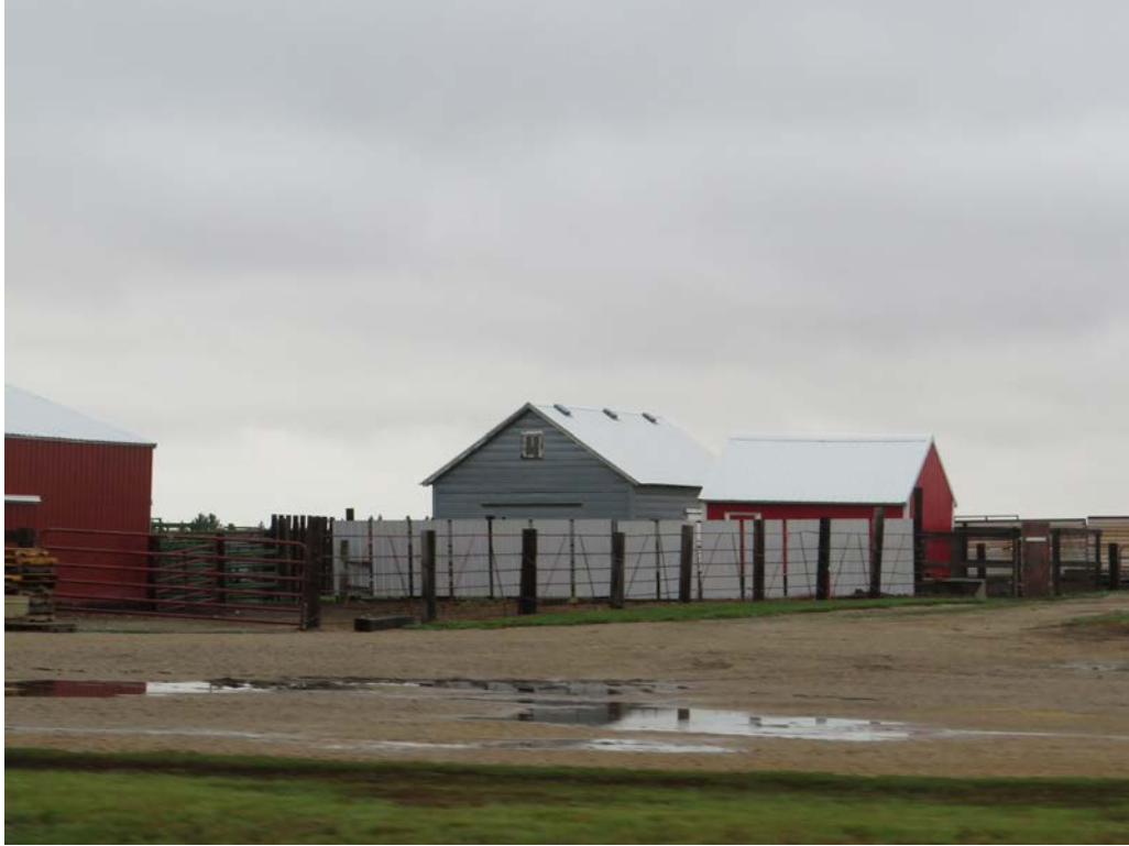
HS-KS-060. 14437 69th St NW, Williston, Williams County, North Dakota. Property overview. View to the Northwest. Photo Number 0760. (Tetra Tech 2025).
