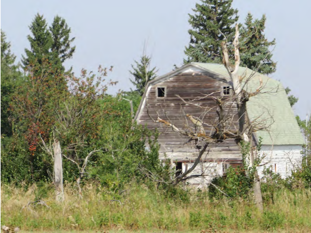
32WIX932. 14606 74th St NW, Grenora, Williams County, North Dakota. F02. View to the Northwest. Photo Number 0480. (Tetra Tech 2025).
