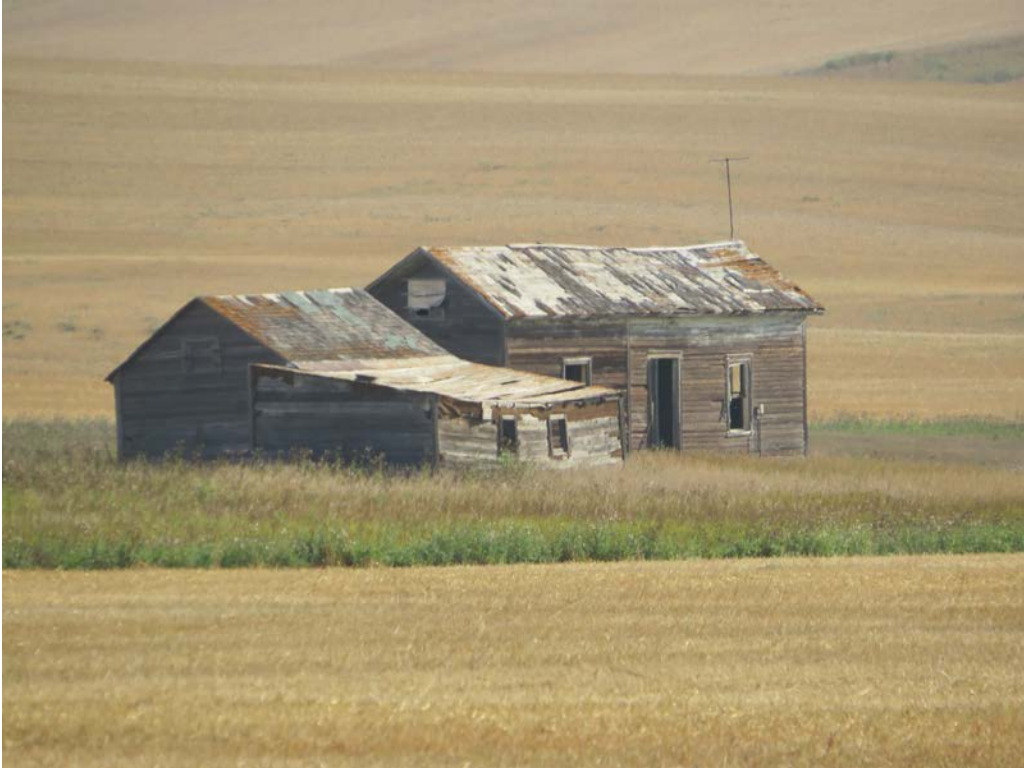
HS-KS-024. 149th Ave NW, Williston, Williams County, North Dakota. Property overview. View to the Northeast. Photo Number 0297. (Tetra Tech 2025).
