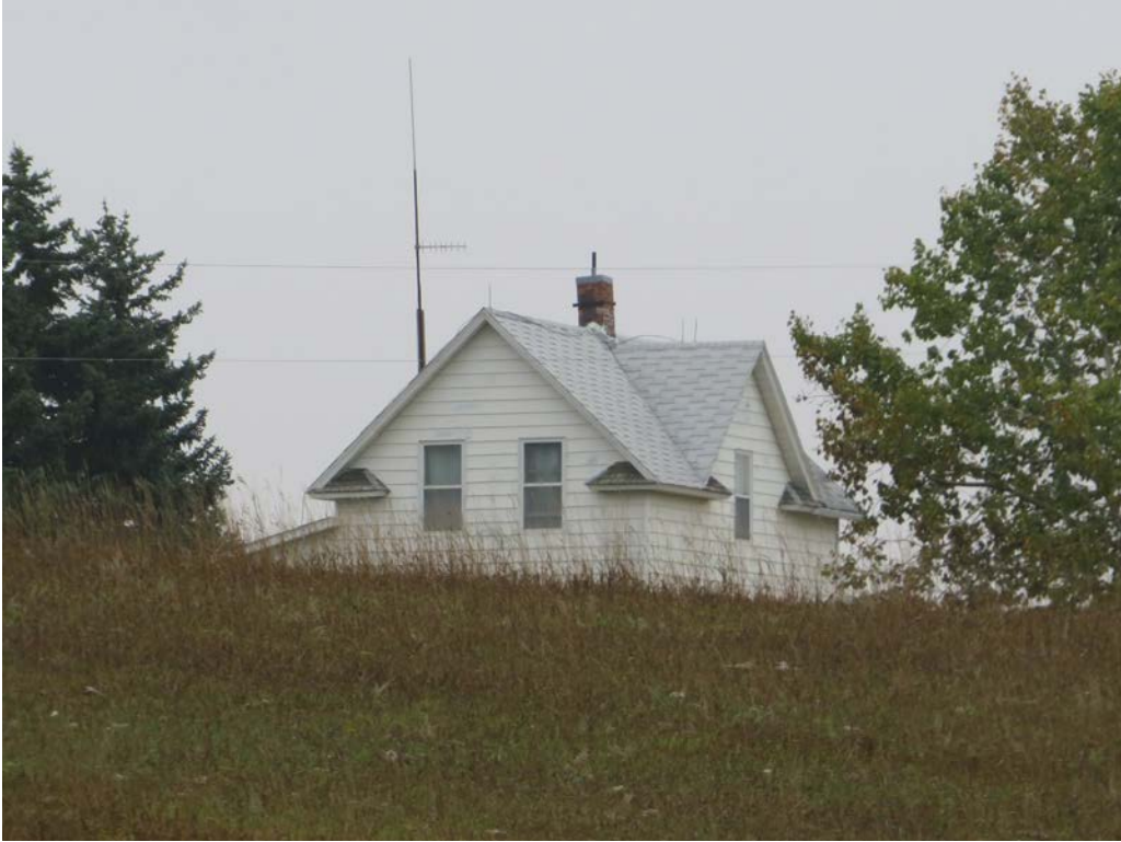
HS-KS-050. 7054 150th Ave NW, Grenora, Williams County, North Dakota. Property overview. View to the Northeast. Photo Number 0673. (Tetra Tech 2025).
