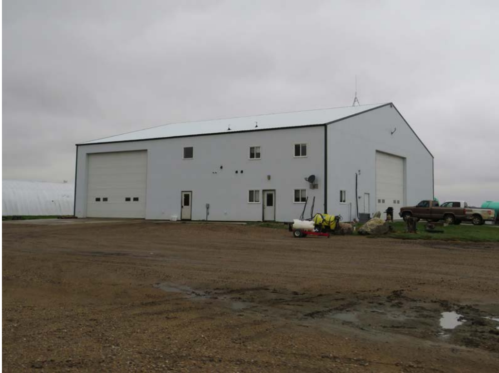
HS-KS-059. 71st St NW, Williston, Williams County, North Dakota. Property overview. View to the North. Photo Number 0751. (Tetra Tech 2025).
