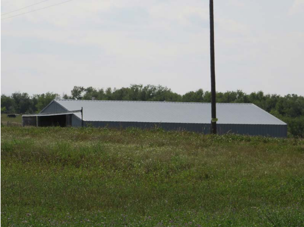
HS-KS-038. 14791 77th St NW, Grenora, Williams County, North Dakota. Property overview. View to the Southeast. Photo Number 0536. (Tetra Tech 2025).
