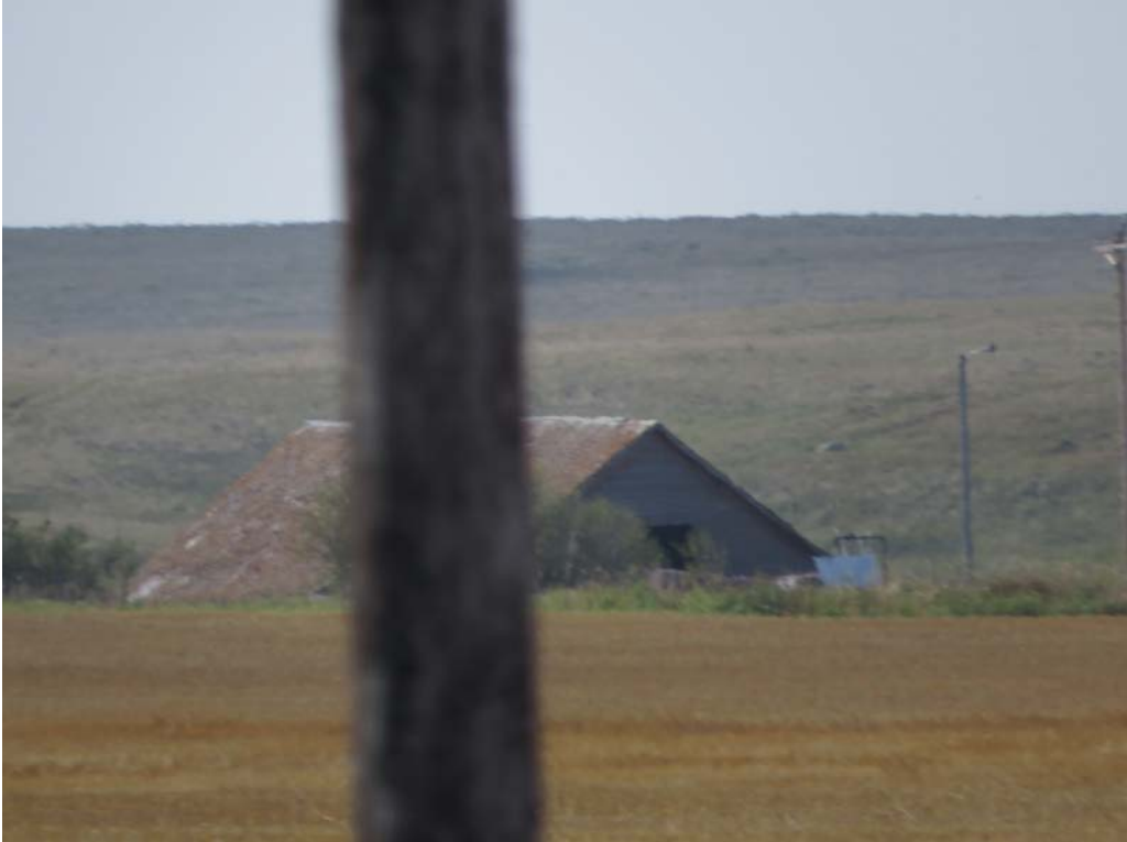
HS-KS-011. 7609 147th Ave NW, Grenora, Williams County, North Dakota. Property overview. View to the Southwest. Photo Number 0137. (Tetra Tech 2025).
