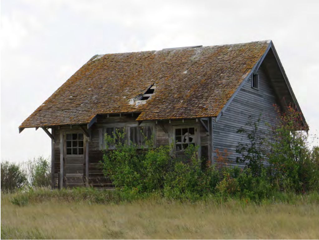
32WIX2458. Eureka Number 2 School.7671-7681 143rd Ave NW, Zahl, Williams County, North Dakota. F01. View to the South-west. Photo Number 0549. (Tetra Tech 2025).
