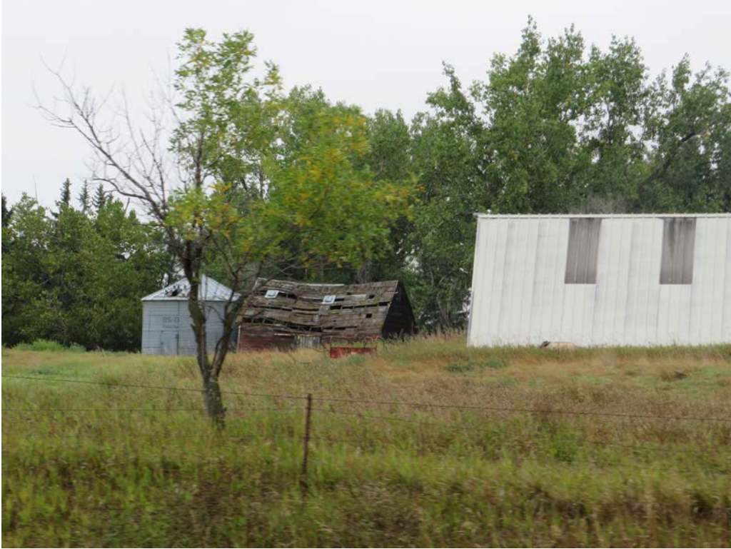
HS-KS-061. 14581 69th St NW, Williston, Williams County, North Dakota. Property overview. View to the North. Photo Number 0777. (Tetra Tech 2025).
