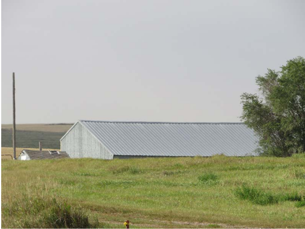
HS-KS-028. 14802 - 14788 67 th St NW, Williston, Williams County, North Dakota. Property overview. View to the Southwest. Photo Number 0377. (Tetra Tech 2025).
