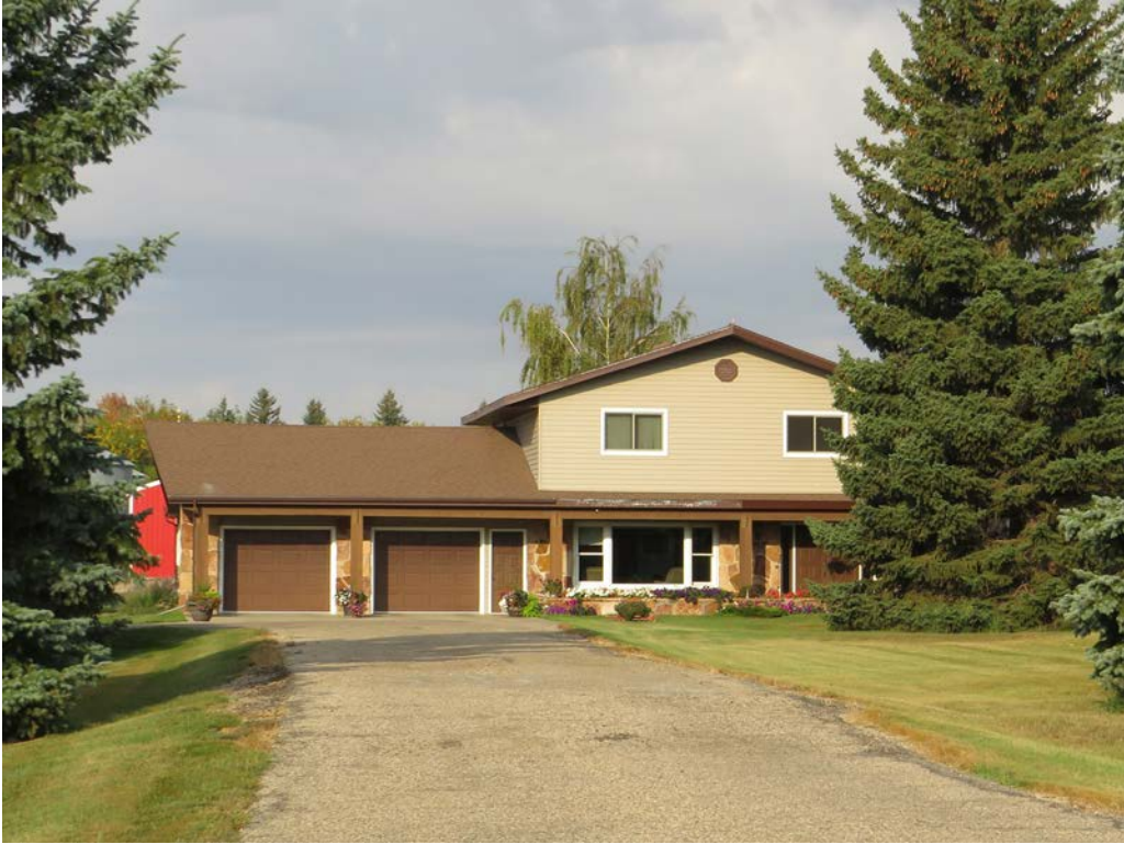
HS-KS-018. 6887 151st Ave NW, Grenora, Williams County, North Dakota. Property overview. View to the West. Photo Number 0224. (Tetra Tech 2025).
