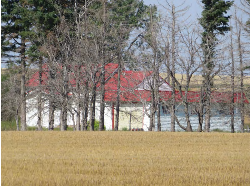
32WIX775. 7053 147th Ave NW, Grenora, Williams County, North Dakota. F01. View to the Northwest. Photo Number 0198. (Tetra Tech 2025).
