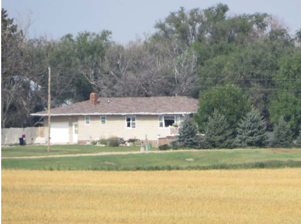
HS-KS-036. 14501 145th Ave NW, Grenora, Williams County, North Dakota. Property overview. View to the Northwest. Photo Number 0502. (Tetra Tech 2025).
