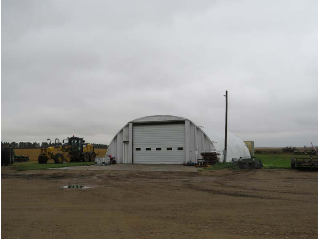
HS-KS-059. 71st St NW, Williston, Williams County, North Dakota. Property overview. View to the North. Photo Number 0753. (Tetra Tech 2025).
