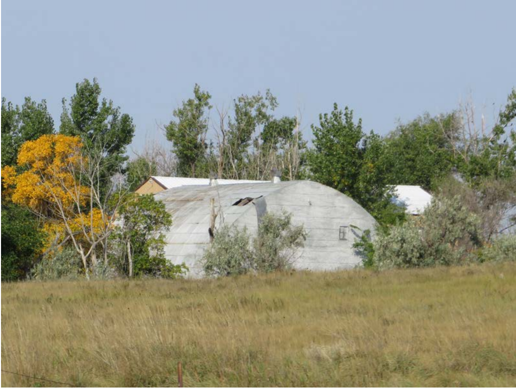
HS-KS-005. 14729 69th St NW, Williston, Williams County, North Dakota. Property overview. View to the Northwest. Photo Number 0052. (Tetra Tech 2025).
