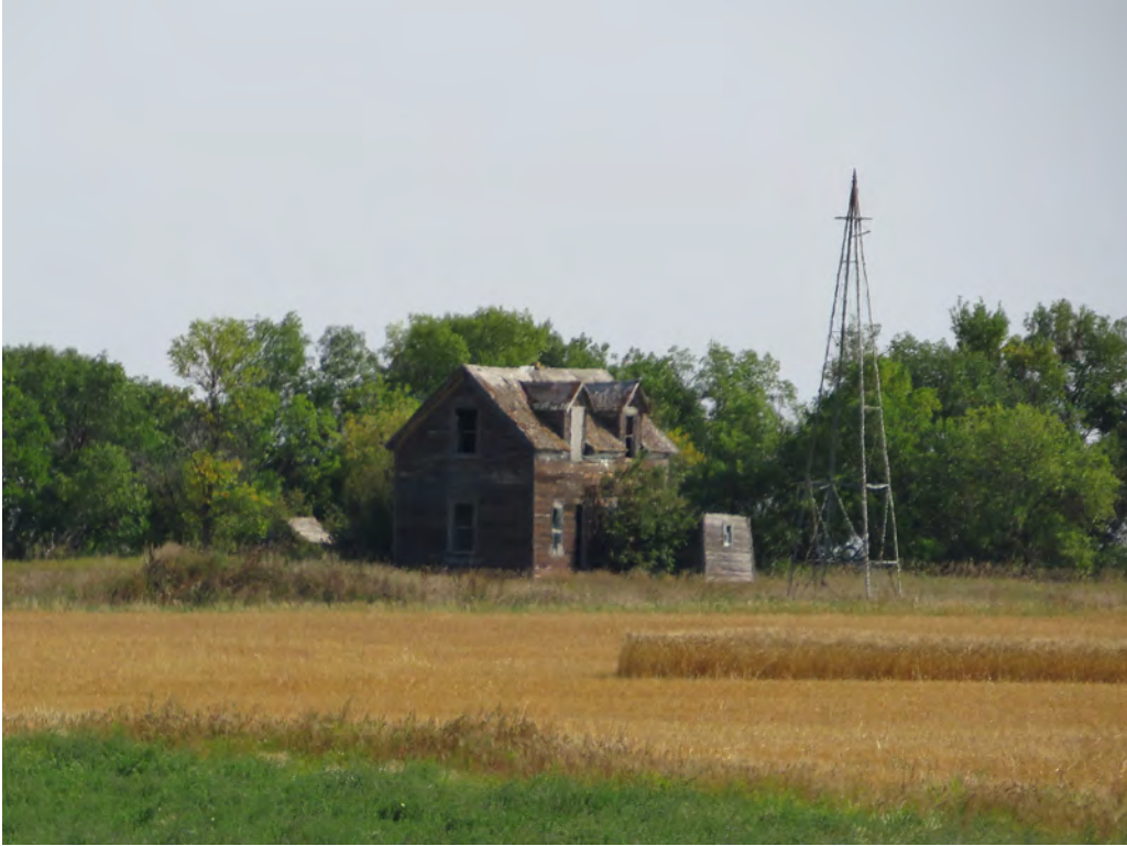
32WI2593. 69th St NW, Grenora, Williams County, North Dakota. F01 (left) and F02 (right). View to the Northeast. Photo Number 0106. (Tetra Tech 2025).
