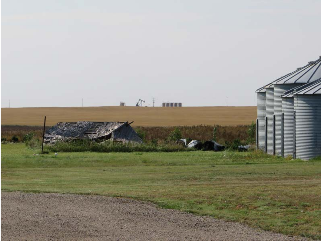
HS-KS-008. 14782 69th St NW, Williston, Williams County, North Dakota. Property overview. View to the Southeast. Photo Number 0110. (Tetra Tech 2025).
