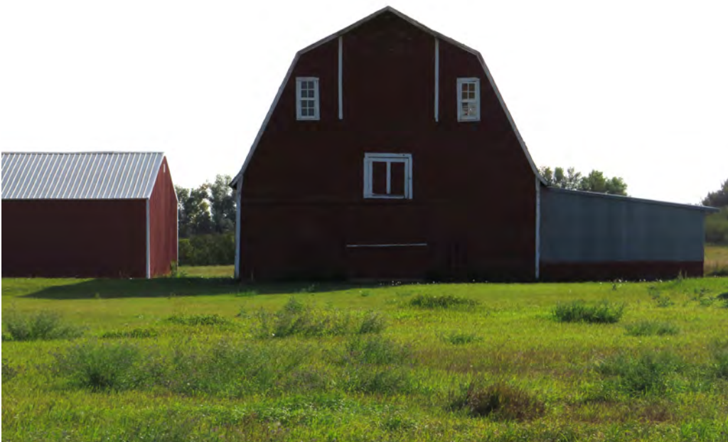
32WIX929. 6894 146th Ave NW, Williston, Williams County, North Dakota. F04 (left) and F02 (right). View to the East. Photo Number 0041. (Tetra Tech 2025).
