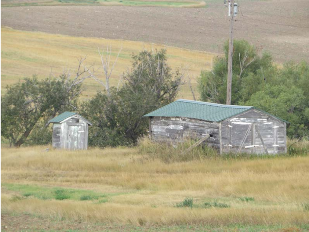
HS-KS-027. 150th Ave NW, Williston, Williams County, North Dakota. Property overview. View to the Northwest. Photo Number 0357. (Tetra Tech 2025).
