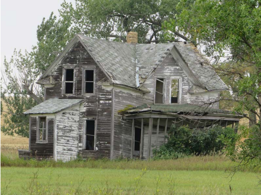
HS-KS-053. 70th St NW, Grenora, Williams County, North Dakota. Property overview. View to the Southwest. Photo Number 0701. (Tetra Tech 2025).
