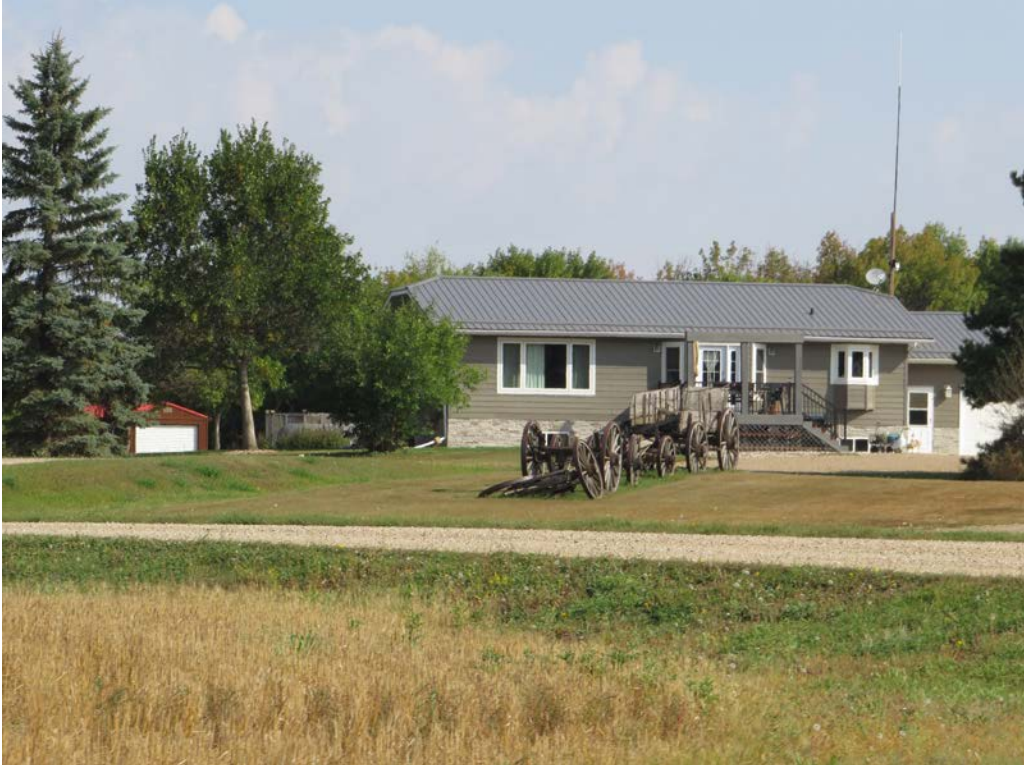
HS-KS-030. 15089 68th St NW, Grenora, Williams County, North Dakota. Property overview. View to the Northeast. Photo Number 0403. (Tetra Tech 2025).
