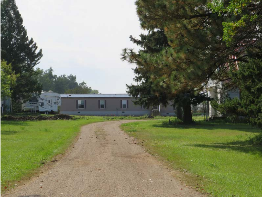
HS-KS-033. 14710 74th st NW, Grenora, Williams County, North Dakota. Property overview. View to the South. Photo Number 0447. (Tetra Tech 2025).
