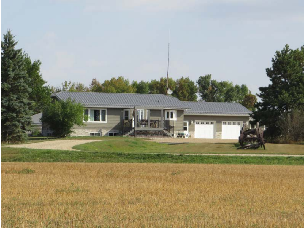
HS-KS-030. 15089 68th St NW, Grenora, Williams County, North Dakota. Property overview. View to the Northeast. Photo Number 0405. (Tetra Tech 2025).
