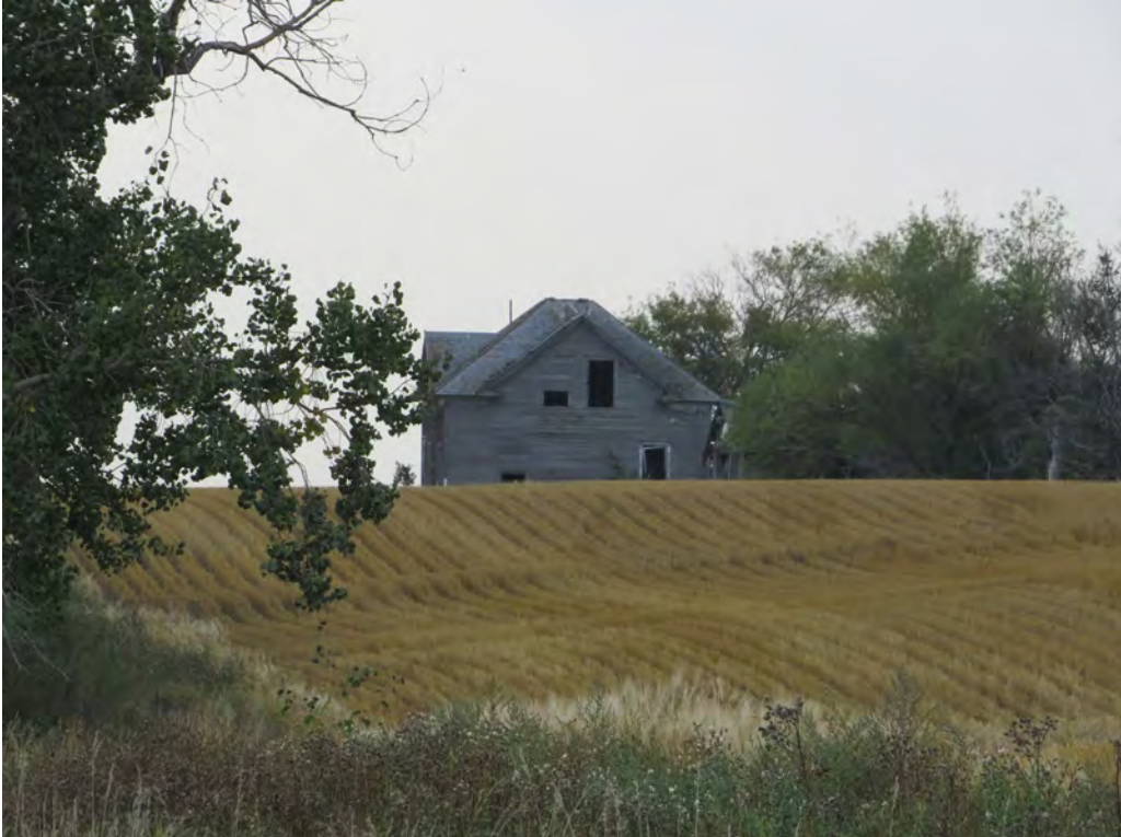
32WIX931. 15024 68th St NW, Williston, Williams County, North Dakota. Property overview. View to the South. Photo Number 0255. (Tetra Tech 2025).
