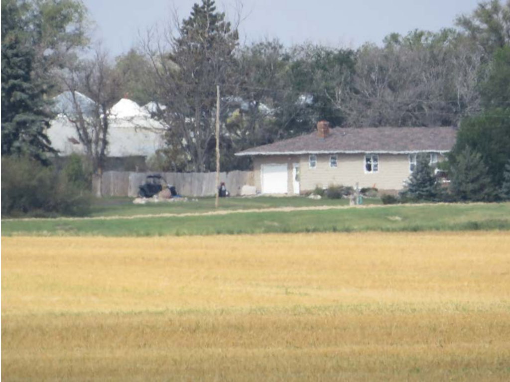
HS-KS-036. 14501 145th Ave NW, Grenora, Williams County, North Dakota. Property overview. View to the Northwest. Photo Number 0498. (Tetra Tech 2025).
