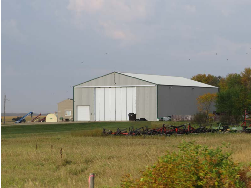
HS-KS-019. 6849 151st Ave NW, Grenora, Williams County, North Dakota. Property overview. View to the Southwest. Photo Number 0238. (Tetra Tech 2025).
