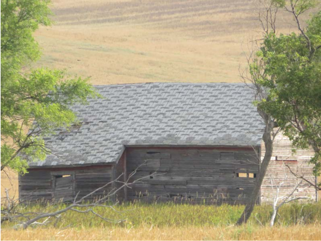
HS-KS-025. 65th St NW, Williston, Williams County, North Dakota. Property overview. View to the Northeast. Photo Number 0330. (Tetra Tech 2025).
