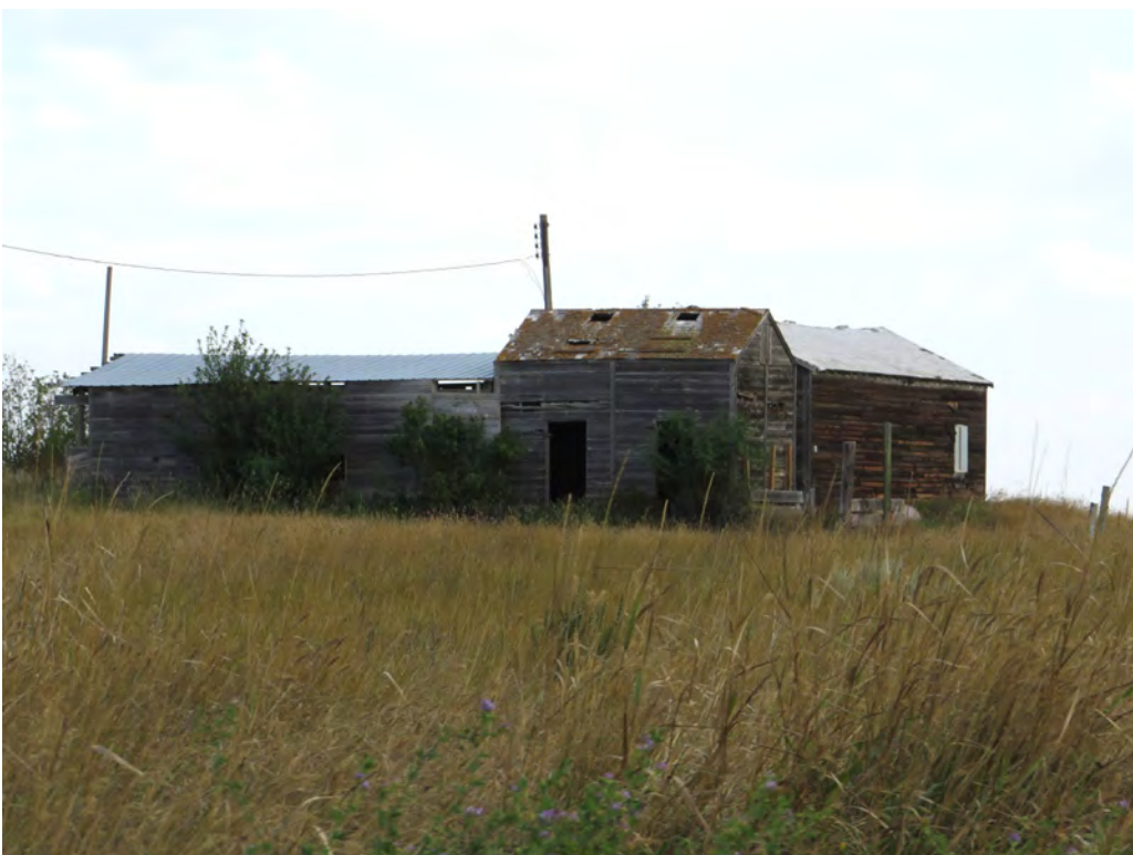
32WI247. 7642 143rd Ave NW, Zahl, Williams County, North Dakota. F03 (right), F04 (left), and F05 (center). View to the Northeast. Photo Number 0562. (Tetra Tech 2025).
