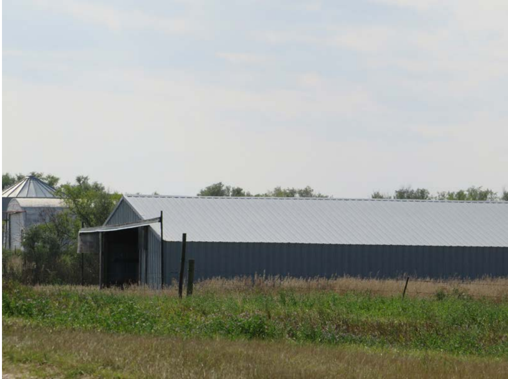
HS-KS-038. 14791 77th St NW, Grenora, Williams County, North Dakota. Property overview. View to the Southeast. Photo Number 0533. (Tetra Tech 2025).
