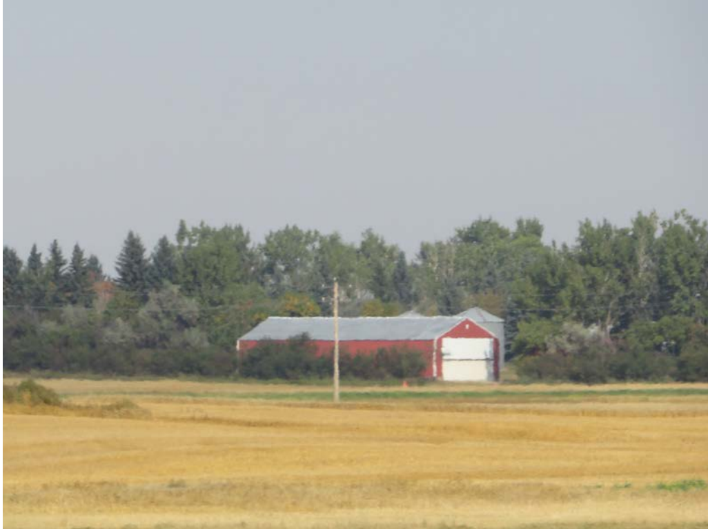
HS-KS-030. 15089 68th St NW, Grenora, Williams County, North Dakota. Property overview. View to the Northwest. Photo Number 0394. (Tetra Tech 2025).
