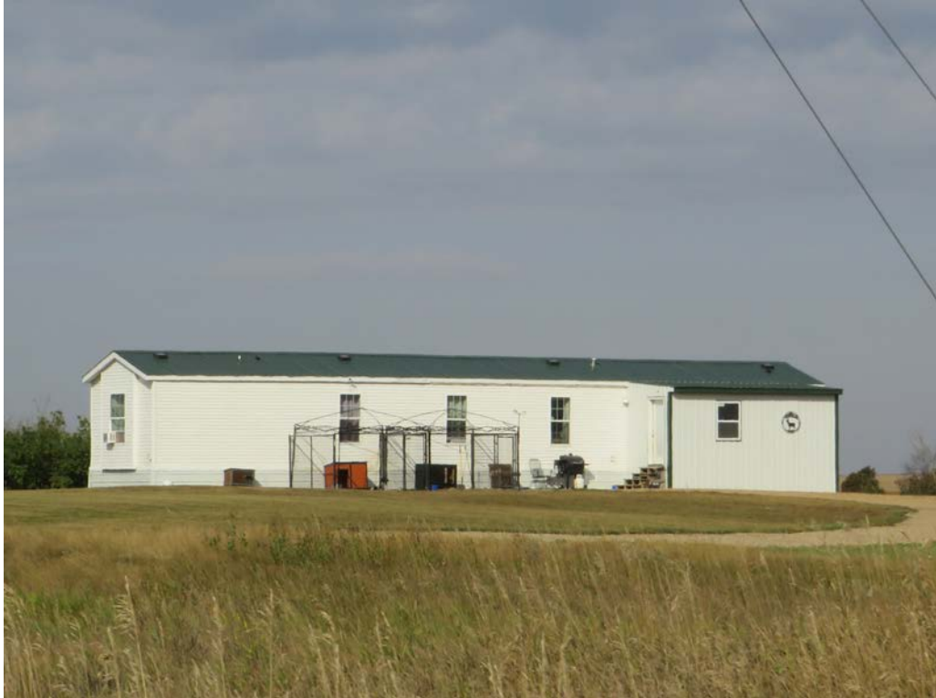
HS-KS-029. 15029 68th St NW, Williston, Williams County, North Dakota. Property overview. View to the Northwest. Photo Number 0382. (Tetra Tech 2025).
