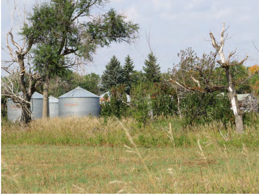
32WIX932. 14606 74th St NW, Grenora, Williams County, North Dakota. F06 (right) and F09 (left). View to the Northwest. Photo Number 0475. (Tetra Tech 2025).
