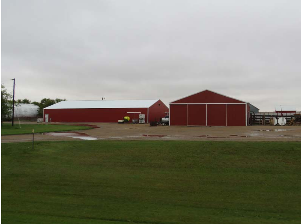
HS-KS-060. 14437 69th St NW, Williston, Williams County, North Dakota. Property overview. View to the North. Photo Number 0762. (Tetra Tech 2025).
