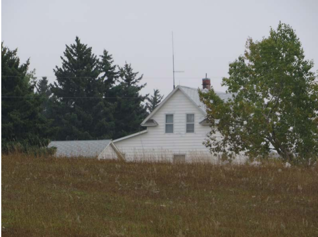
HS-KS-050. 7054 150th Ave NW, Grenora, Williams County, North Dakota. Property overview. View to the Northeast. Photo Number 0672. (Tetra Tech 2025).
