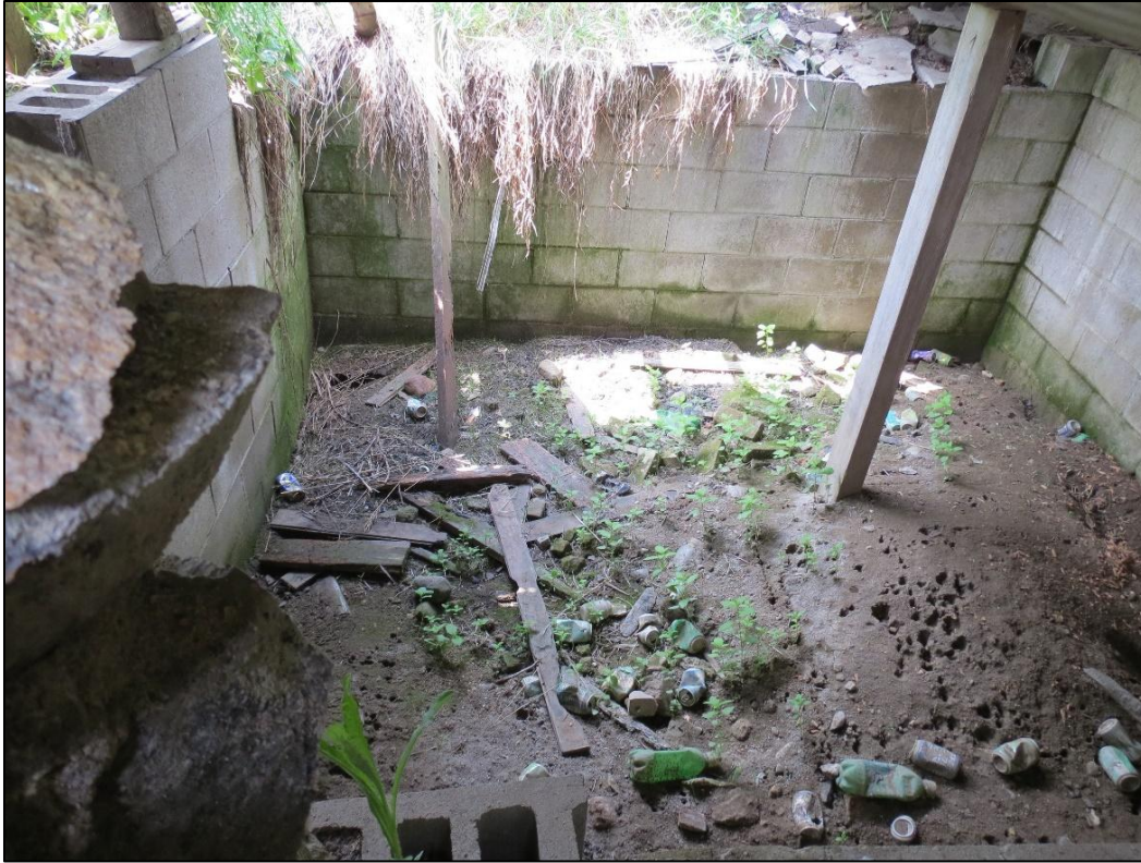
Figure 6-50. Feature 7- House basement at 32WI2607. View looking west.
