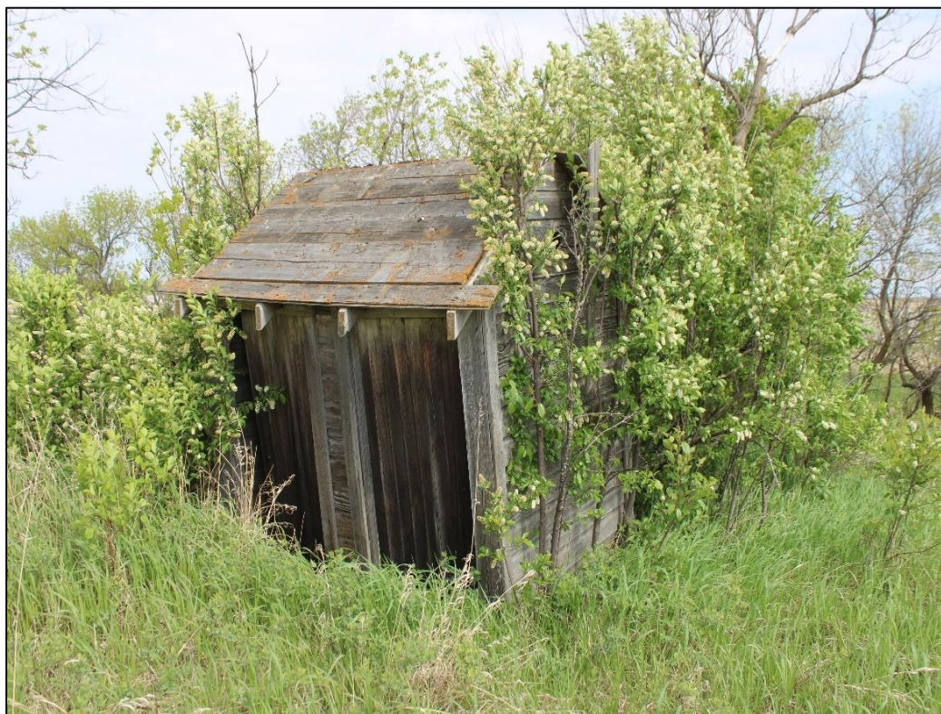
Figure 6-10. Feature 2- Wood framed outhouse at 32WI2593. View looking northwest.
