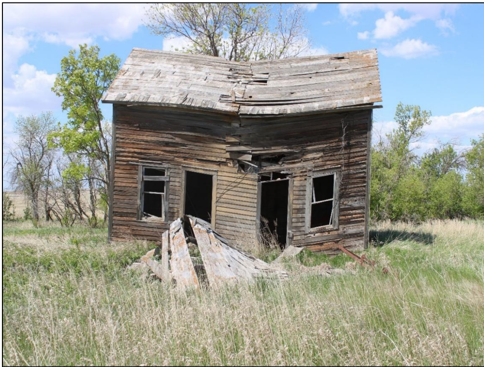
Figure 6-14. Feature 1- Wood farmed house structure at 32WI2594. View looking north.
