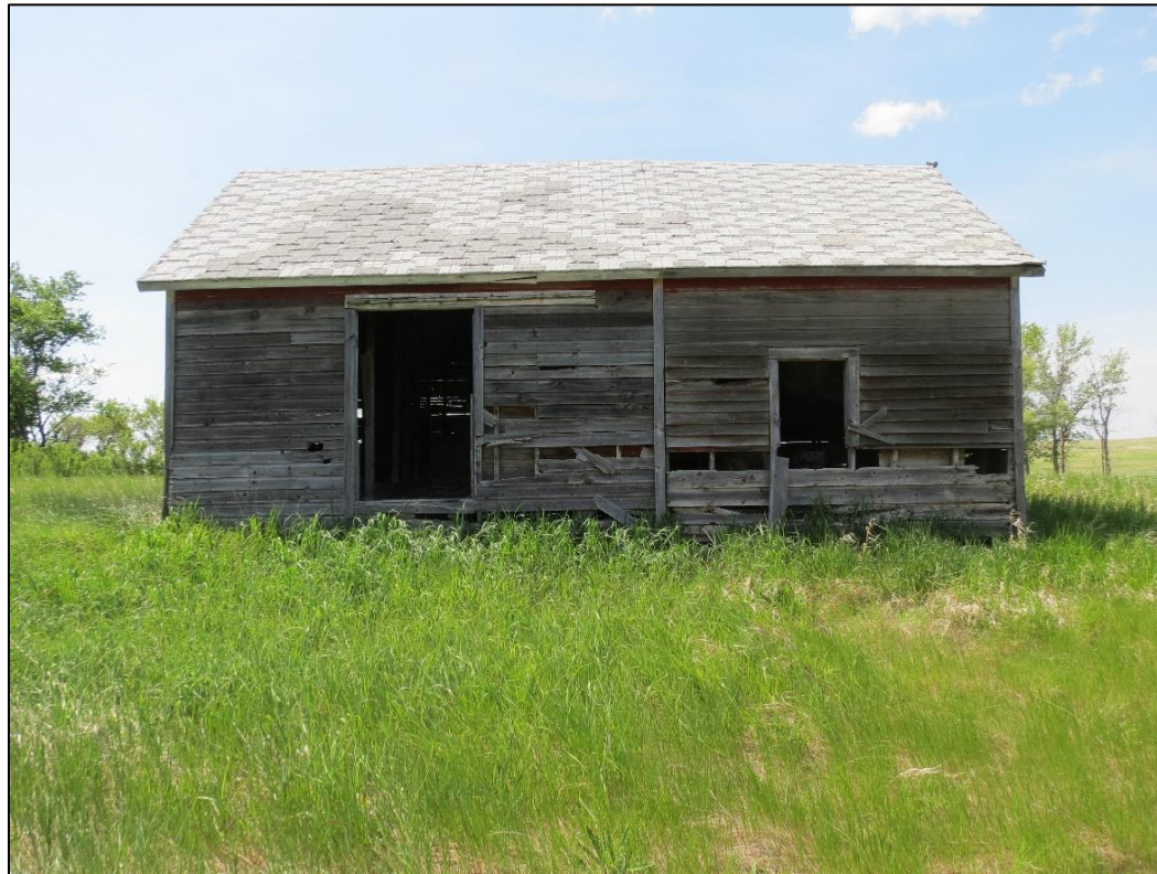
Figure 6-38. Feature 4- Wood framed structure at 32WI2604. View looking west.
