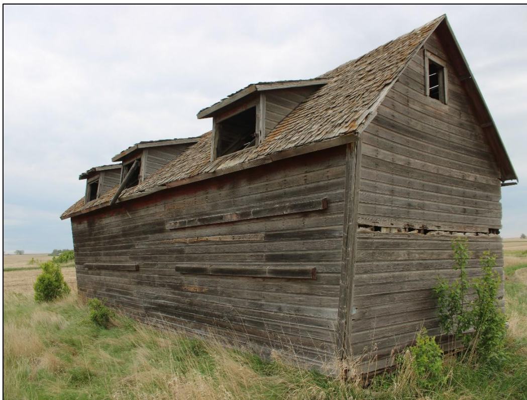
Figure 6-53. Feature 2- Wood framed structure at 32W1148. View looking northwest.
