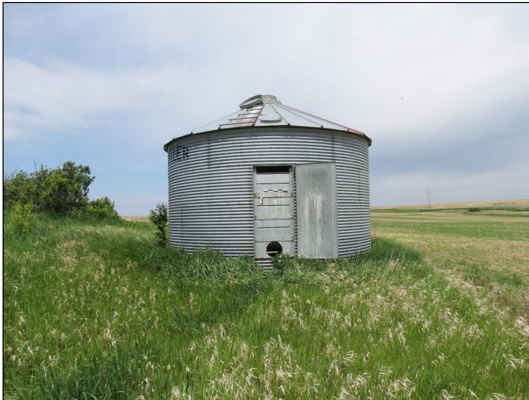
Figure 6-43. Feature 2- Butler corrugated metal silo at 32WI2607. View looking north.
