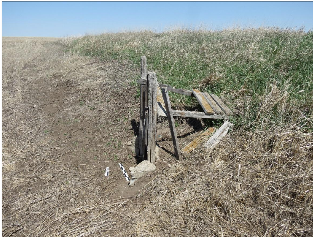
Figure 6-29. Feature 1- Turn out at 32WI2601. View looking north.
