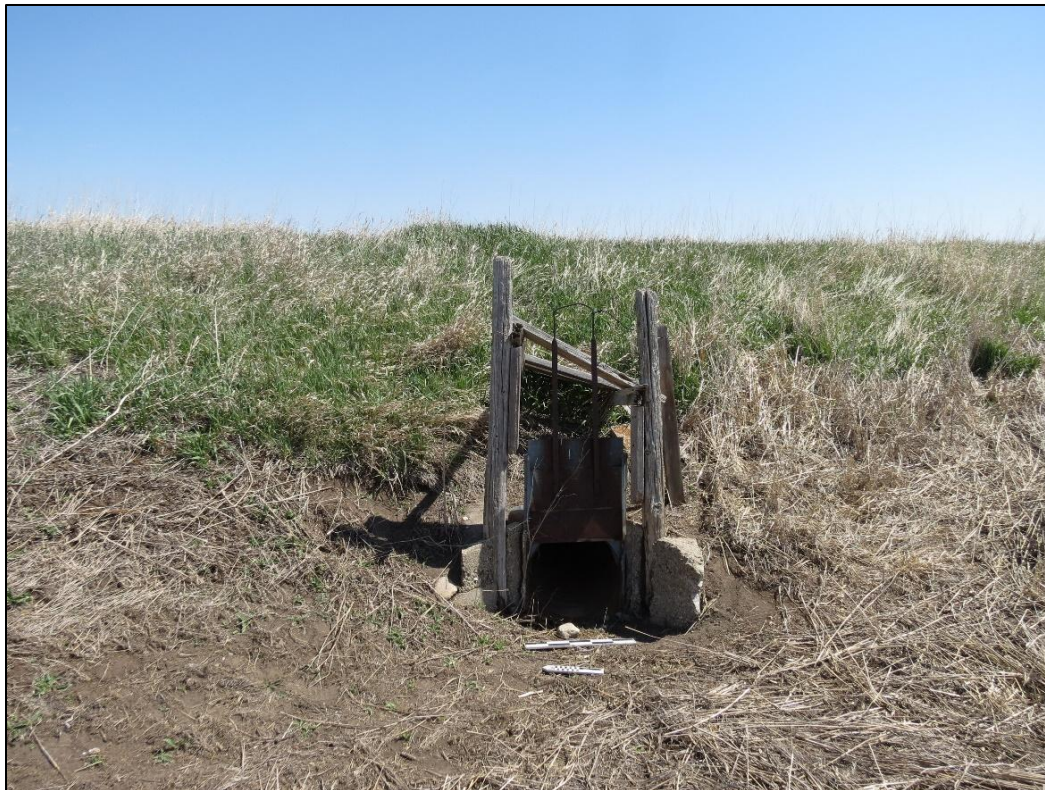
Figure 6-28. Feature 1- Turn out at 32WI2601. View looking east.
