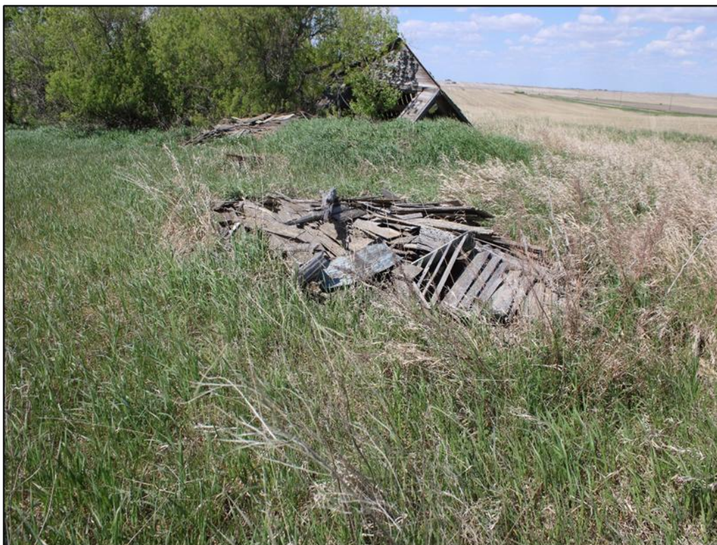
Figure 6-20. Feature 5- Collapsed wood framed outhouse at 32WI2594. View looking north.
