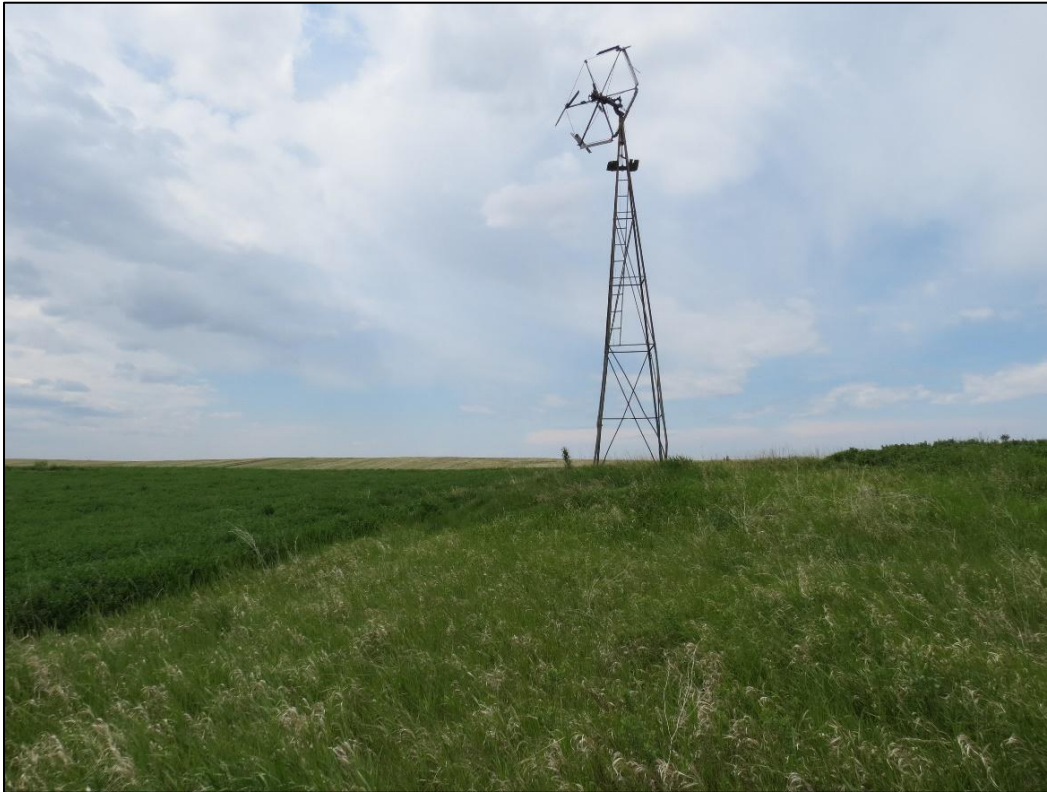
Figure 6-42. Feature 1- Windmill at 32WI2607. View looking west.
