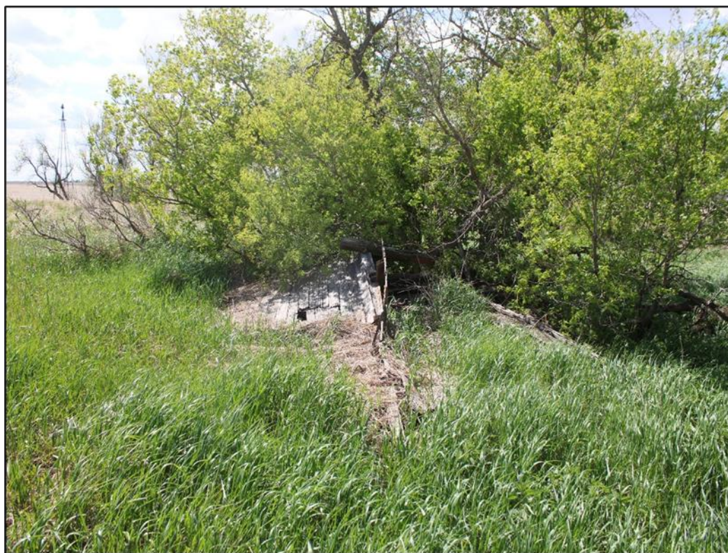
Figure 6-18. Feature 3- Collapsed wood framed structure at 32WI2594. View looking west.
