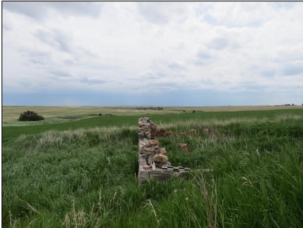
Figure 6-44. Feature 3- Stone and mortar structure at 32WI2607. View looking south.
