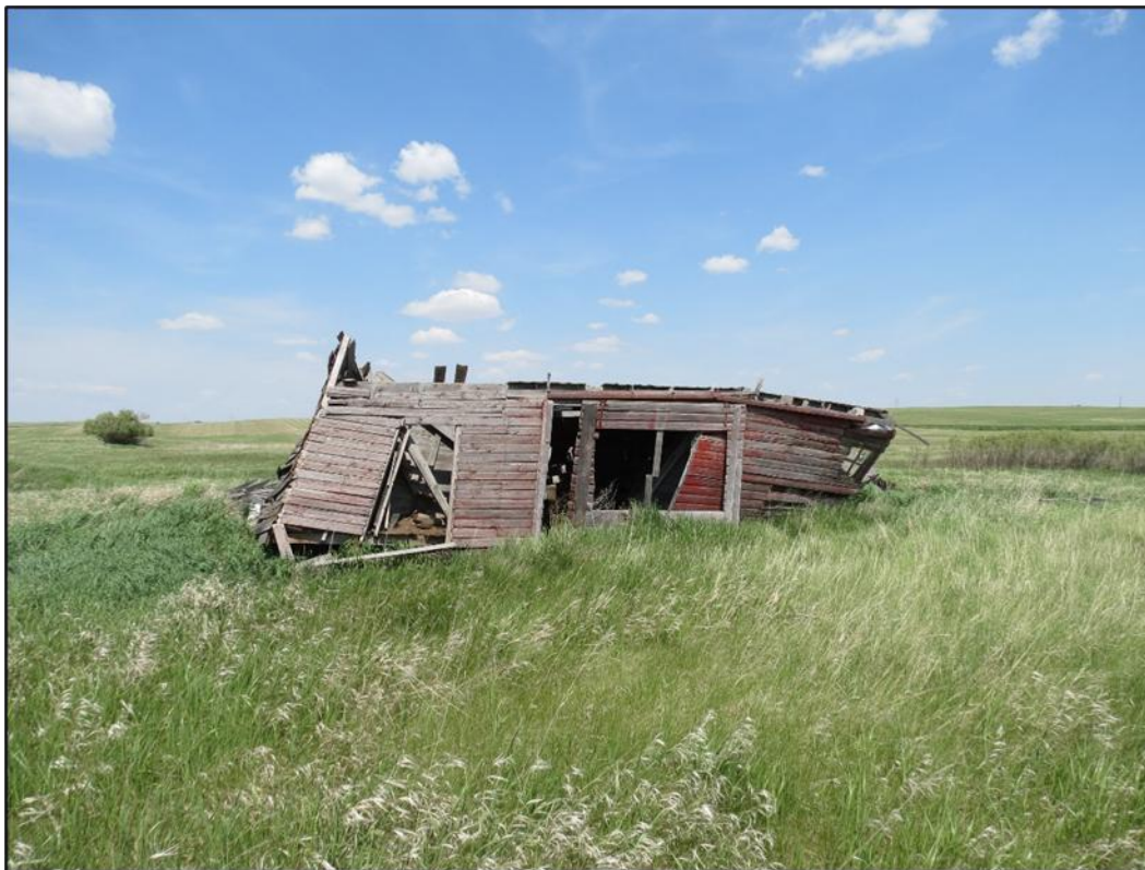
Figure 6-39. Feature 5- Partially collapsed barn at 32WI2604. View looking north.
