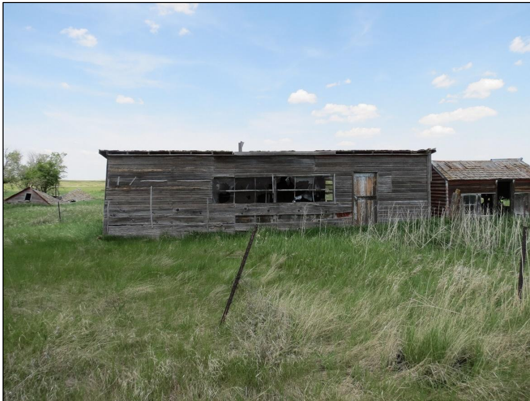
Figure 6-35. Feature 2- Wood framed structure at 32WI2604. View looking north.
