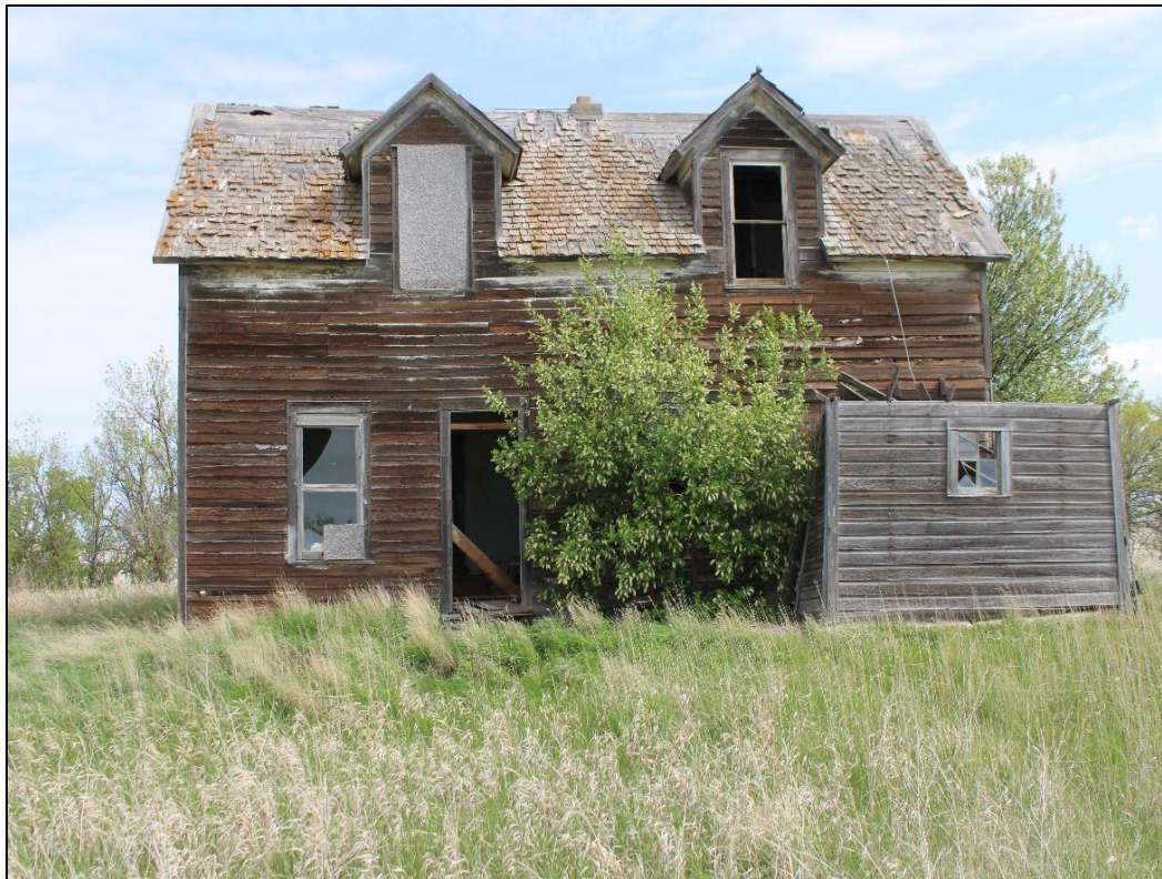
Figure 6-7. Feature 1- Wood framed house at 32WI2593. View looking north.
