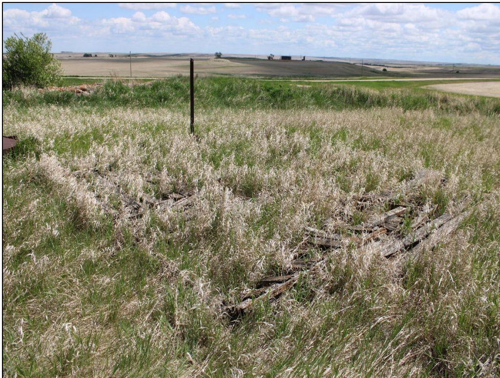
Figure 6-22. Feature 7- Collapsed wood structure at 32WI2594. View looking southwest.
