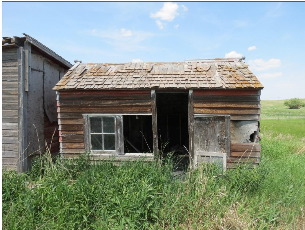
Figure 6-36. Feature 3- Wood framed structure at 32WI2604. View looking north.
