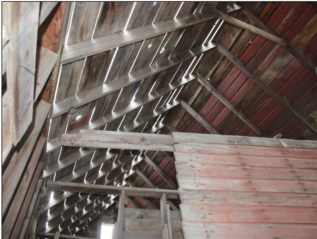
Figure 6-55. Feature 2- Interior of wood framed structure at 32WI1148. View looking southeast.
