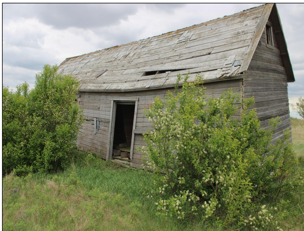
Figure 6-54. Feature 2- Wood framed structure at 32W1148. View looking southeast.
