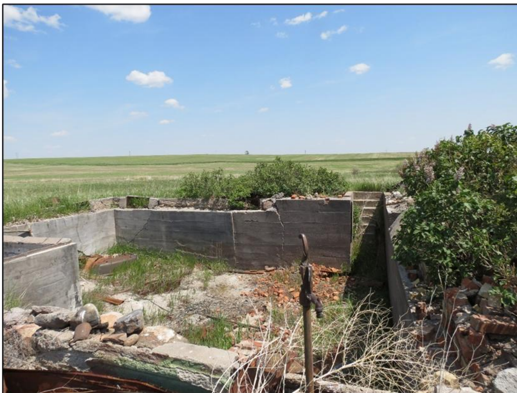
Figure 6-40. Feature 6- Form poured concrete foundation at 32WI2604. View looking east.
