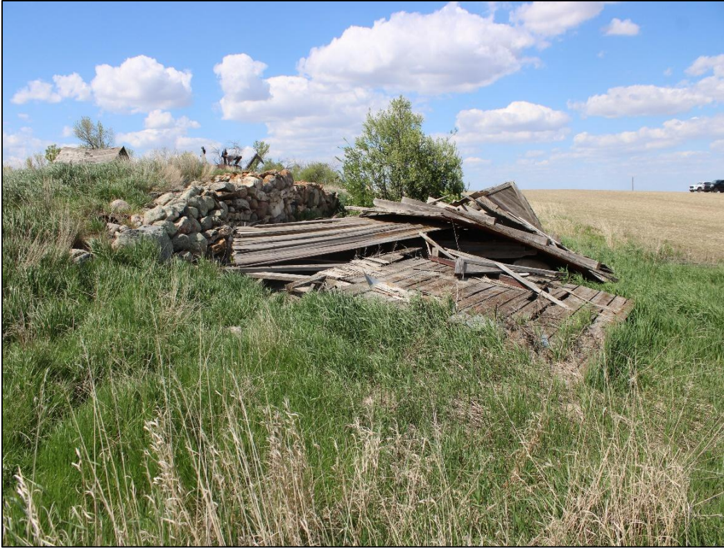
Figure 6-21. Feature 6- Collapsed wood and masonry structure at 32WI2594. View looking north.
