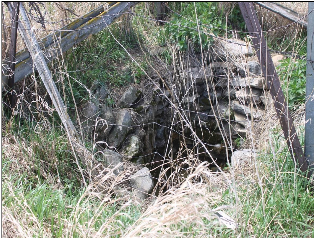
Figure 6-3. Feature 1- Stacked rock-lined well and windmill at 32WI2592. View looking southwest.
