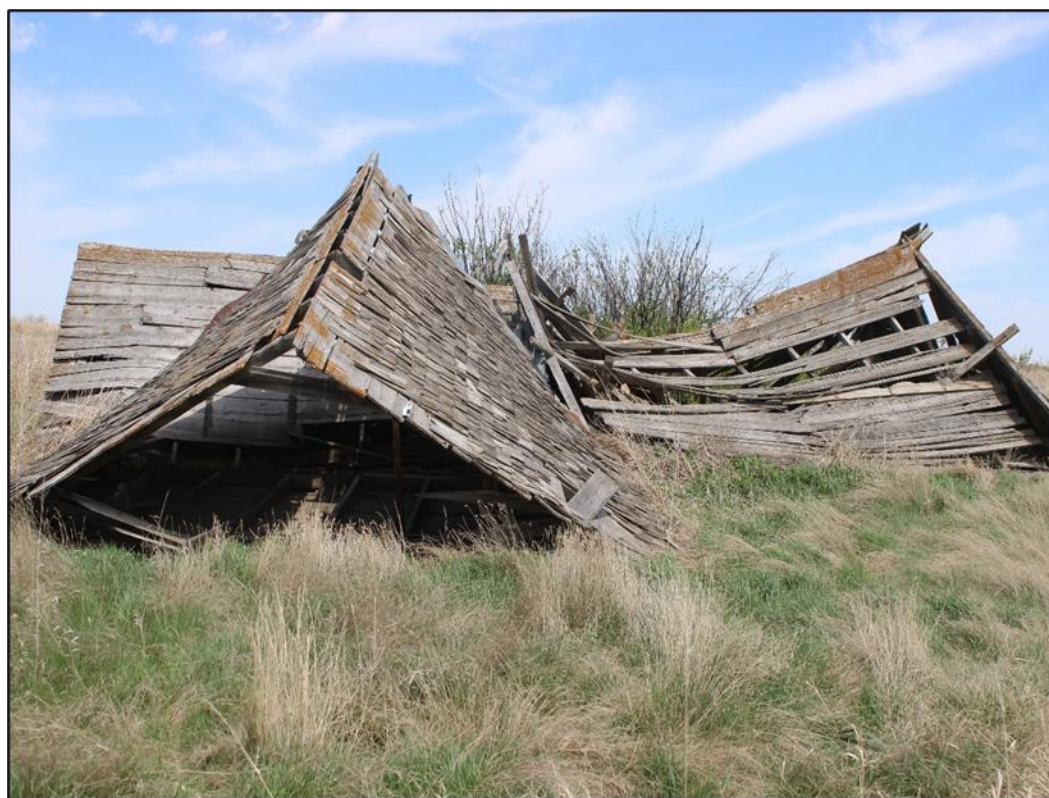
Figure 6-6. Feature 2- Collapsed wood framed house at 32WI2592. View looking southeast.
