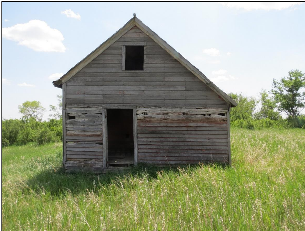
Figure 6-37. Feature 4- Wood framed structure at 32WI2604. View looking south.
