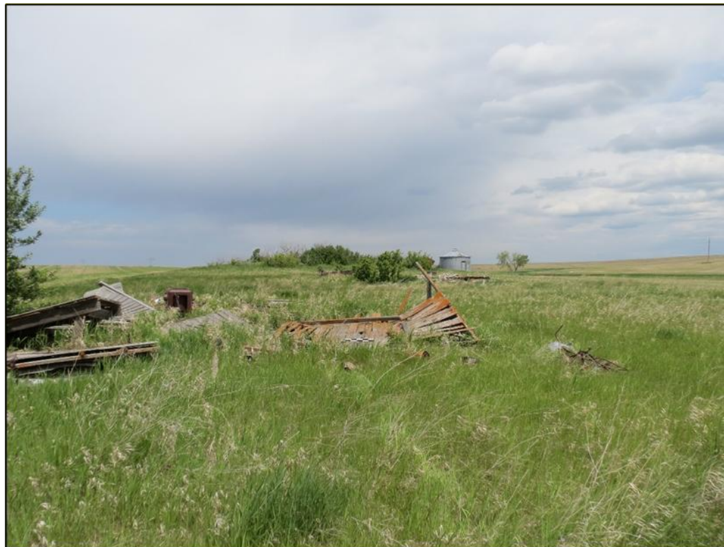
Figure 6-48. Feature 6- Collapsed wood structure at 32WI2607. View looking north.
