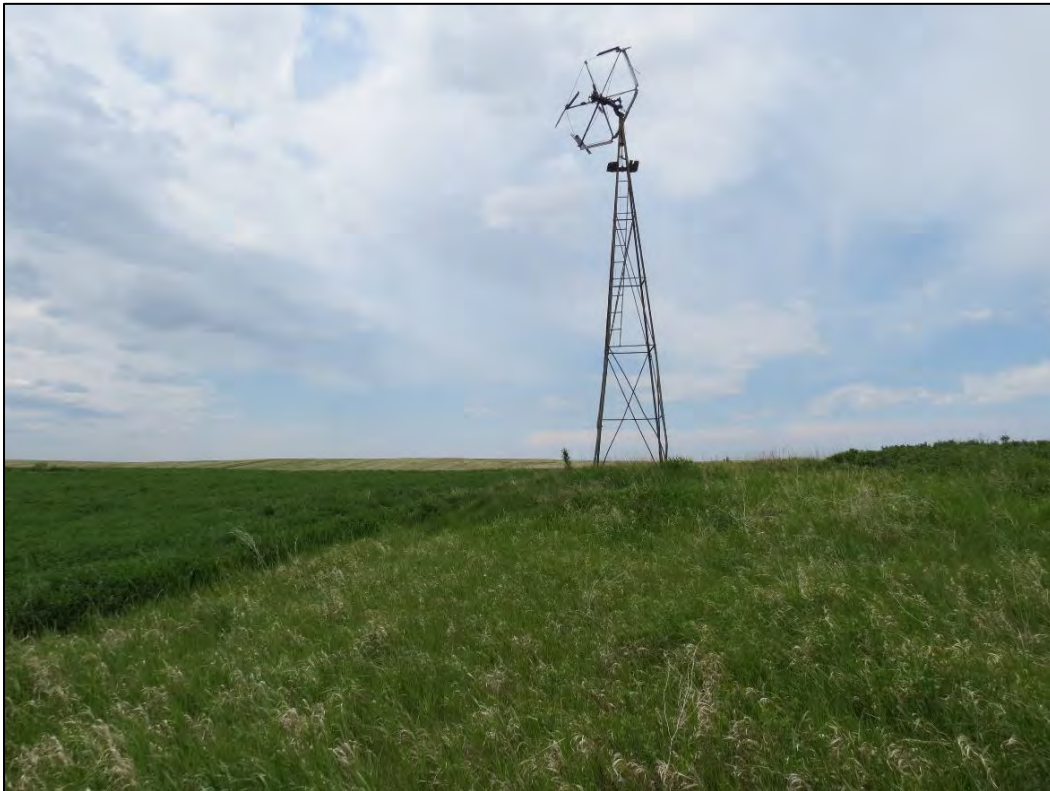
Figure 6-42. Feature 1- Windmill at 32WI2607. View looking west.
