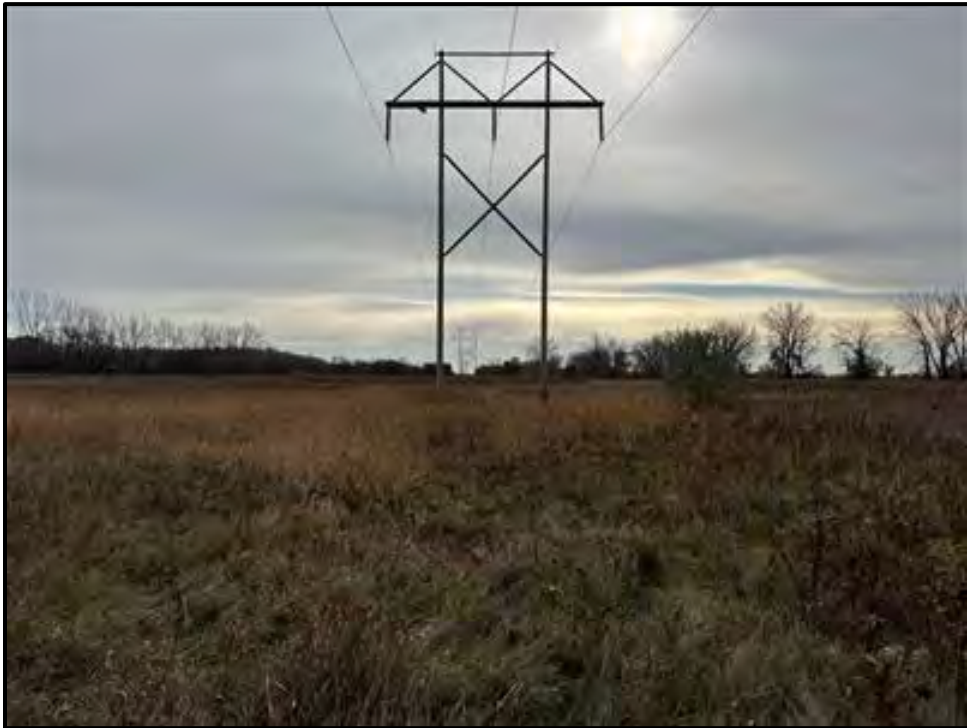
Figure 61: Overview of Study Area 22, Pole 225. View to the southeast.
