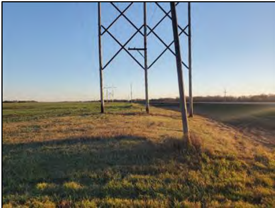
Figure 45: Overview of Study Area 6, Pole 325. View to the south.
