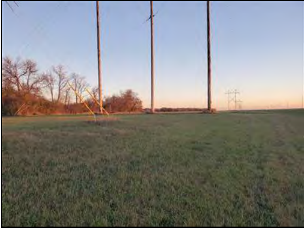
Figure 47: Overview of Study Area 4, Pole 306. View to the south.
