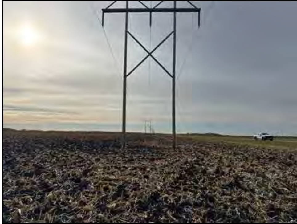
Figure 70: Overview of Study Area 31, Pole 93. View to the south.
