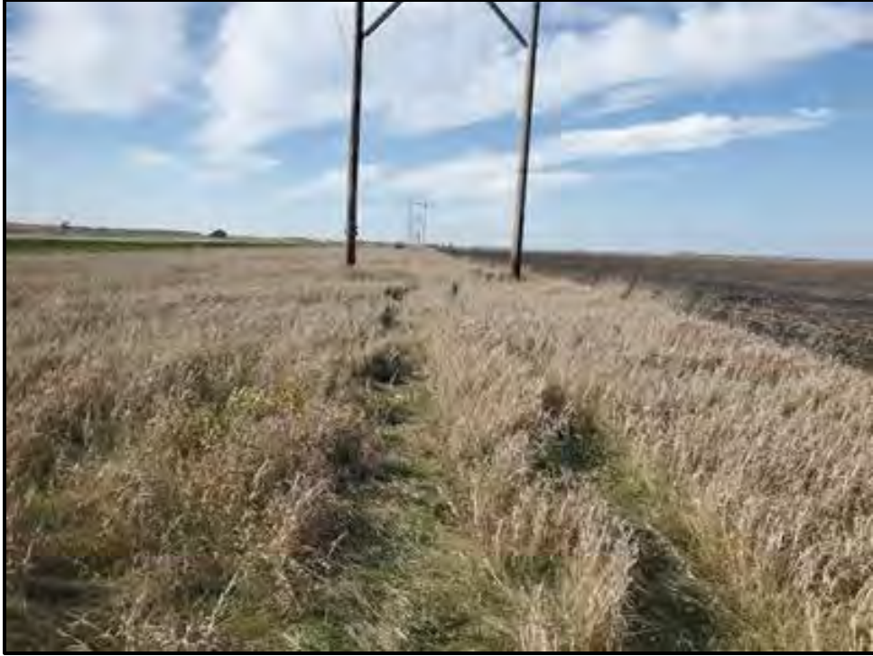
Figure 56: Overview of Study Area 17, Pole 250. View to the west.
