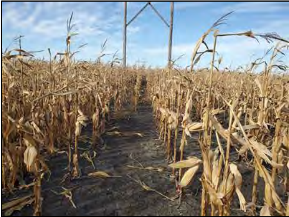
Figure 51: Overview of Study Area 12, Pole 269. View to the west.
