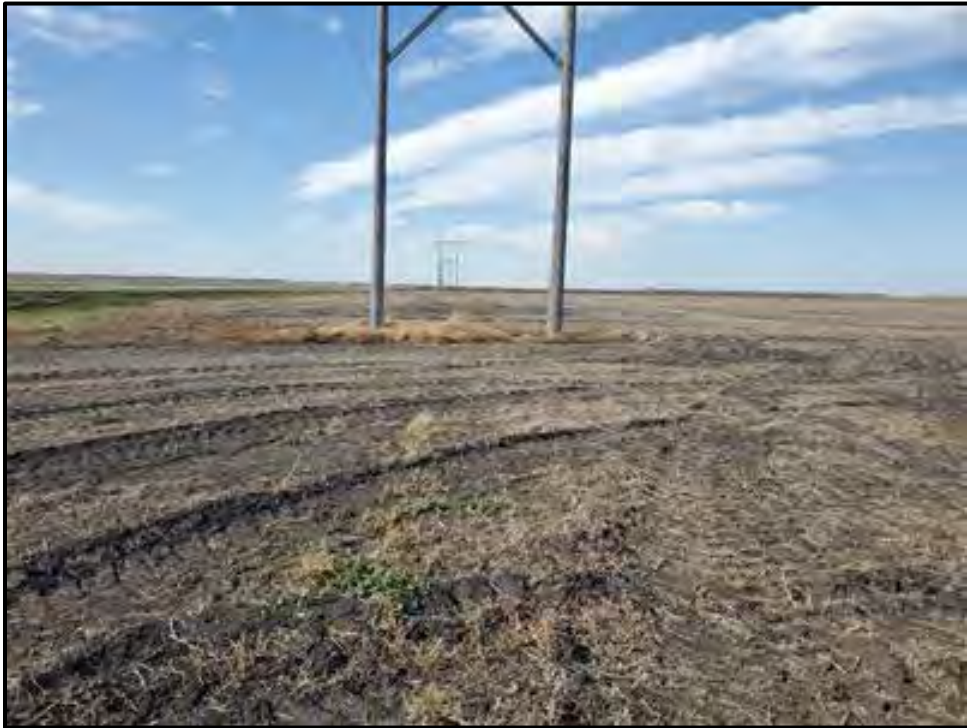
Figure 55: Overview of Study Area 16, Pole 256. View to the west.
