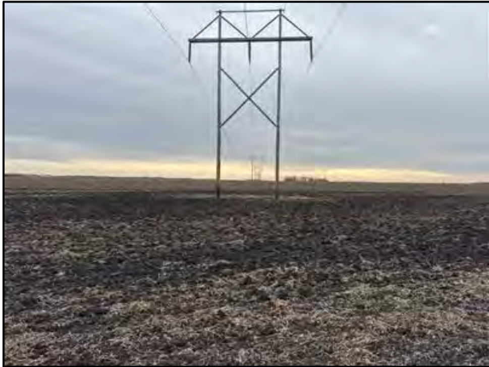
Figure 73: Overview of Study Area 34, Pole 89. View to the south.
