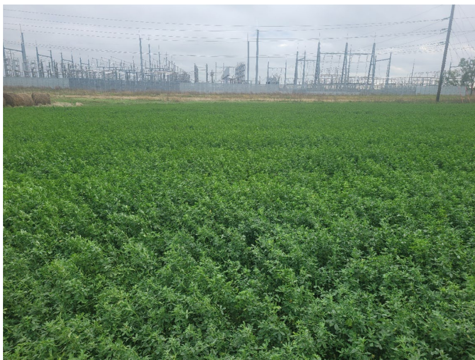
Figure 4: Overview of inventory area from center looking towards current substation, view to the east.
