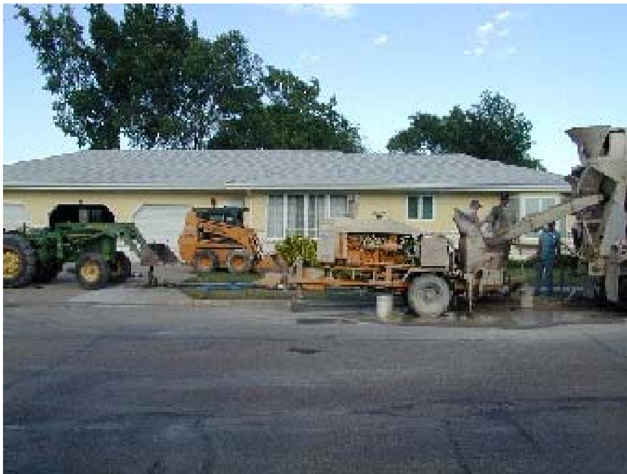
Figure 2: Pressurized grout remote backfilling near the Jack Thielman residence in Beulah.
